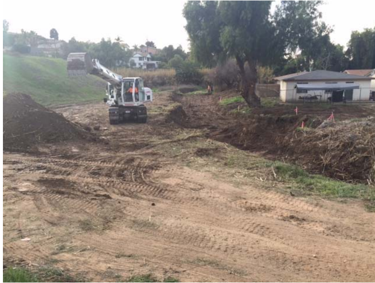
Photograph 7: Photo taken from 69 th St. looking west at the Gradall removing vegetation and sediment from the channel and unloading debris into a temporary stockpile.
