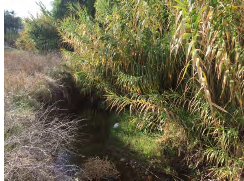
Photograph 4: Looking downstream at the vegetated stream channel that has been constricted by sediment deposits and large stands of Arundo.
