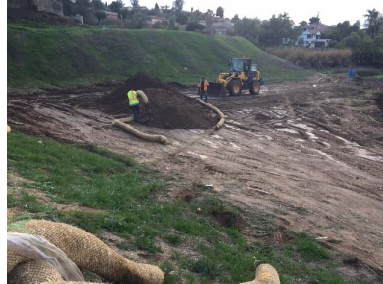
Photograph 8: Photo taken from 69 th St. looking southwest at the BMPs around the stockpile area (i.e. fiber rolls). This material was taken to the Miramar Landfill post-construction.
