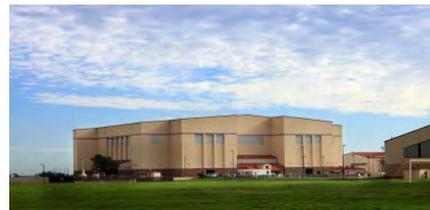
Exterior walls were CMU to 16' and steel superstructure covered with pre-insulated stucco embossed panels with enhanced insulating qualities. Natural daylighting was provided through the use of translucent panels strategically placed to optimize day-lighting. Windows were also included in all regularly occupied spaces to provide views to exterior spaces. In addition to the maintenance bays the facility included two equipment storage bays, private office
