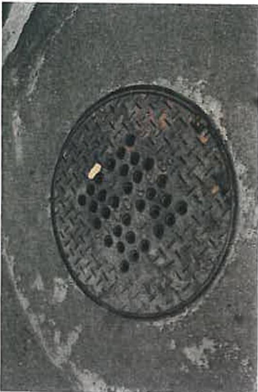
Figure 6: SDG&E manhole cover for underground transformers, Ridgeway, July 2010
