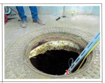
The underside of the top slab is shown here. The bottom layer of rebar is exposed over nearly the entire top slab. The concrete appears to be deteriorated up to approximately the top of the bottom layer of reinforcement. At multiple locations, reinforcement is broken, damaged, or extensively corroded.
