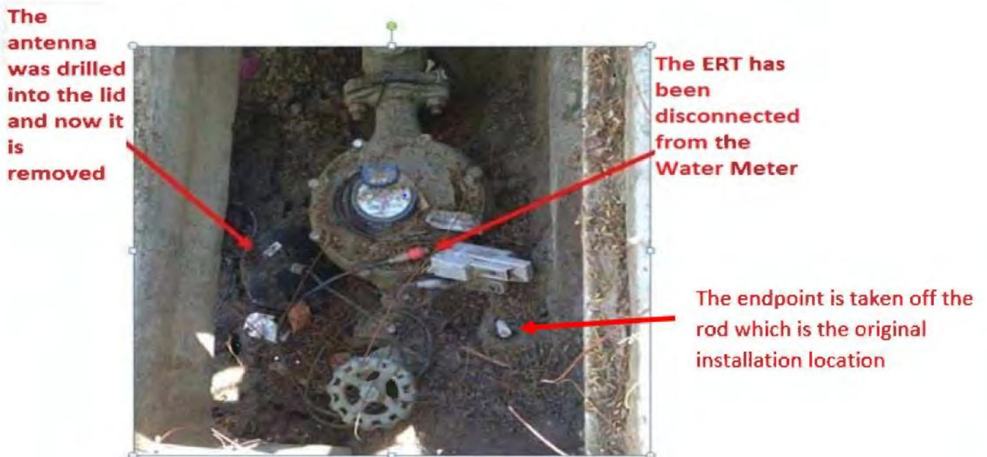
**You are responsible when working in and around meter boxes.** If you encounter these endpoints, use proper care and do not disconnect them from the registers on top of the water meter. If the lid has an antenna drilled through, do not change or tamper with the lid and inform the Resident Engineer immediately about the location of that lid. Refer to Photo 7 below:
