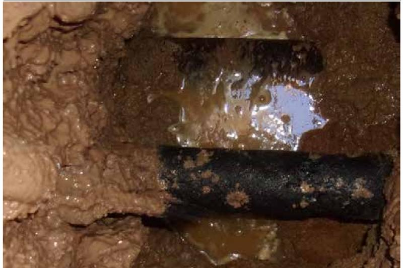
A downhole view of the utilities found in Pothole 15 and their orientation at the pothole location: a 3 inch steel gas utility at the depth of 41 inches T/P and runs in a W/E direction; and a 4 inch PVC electric utility at the depth of 53 inches T/P and runs in a W/E direction. Utilities were found directly on markout.
