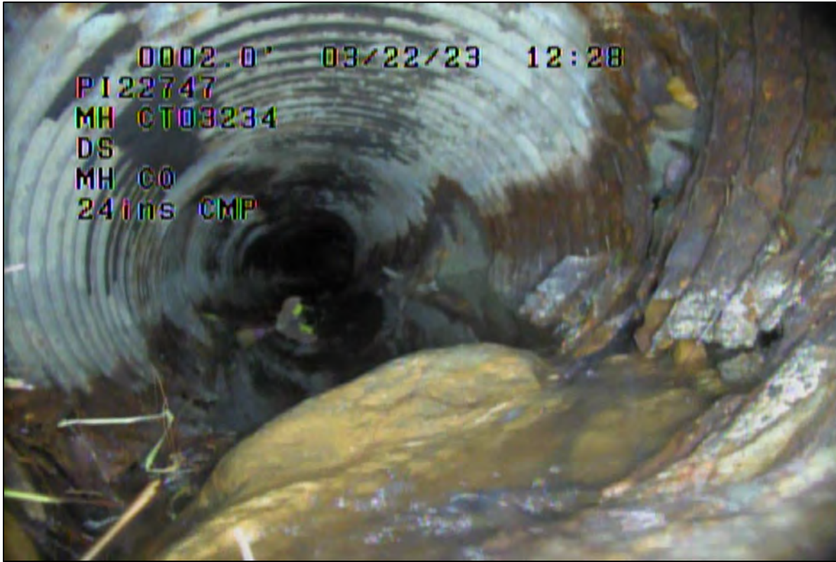
Figure 5 - CCTV of Downstream Pipe from Structure near 5995 Eldergardens Street (3/22/2023)
