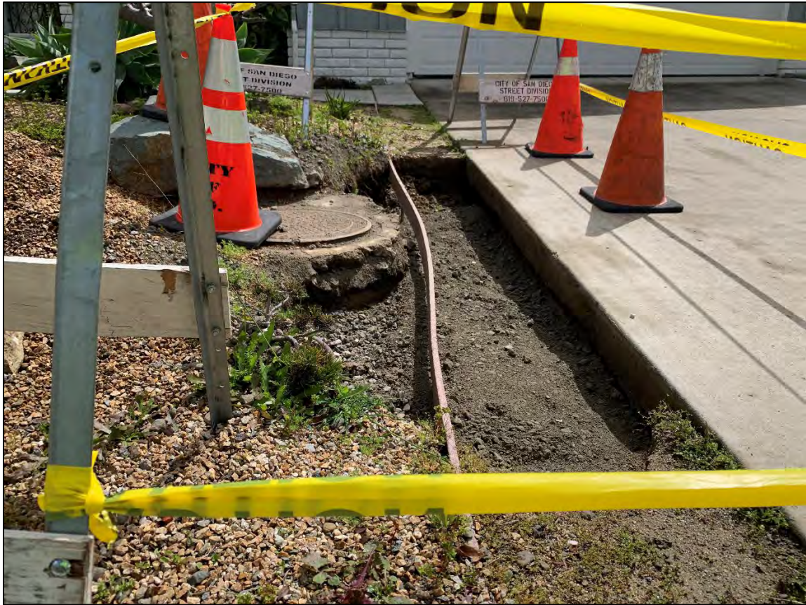
Figure 3 - Field Conditions, Class II backfill in place (3/21/2023)
