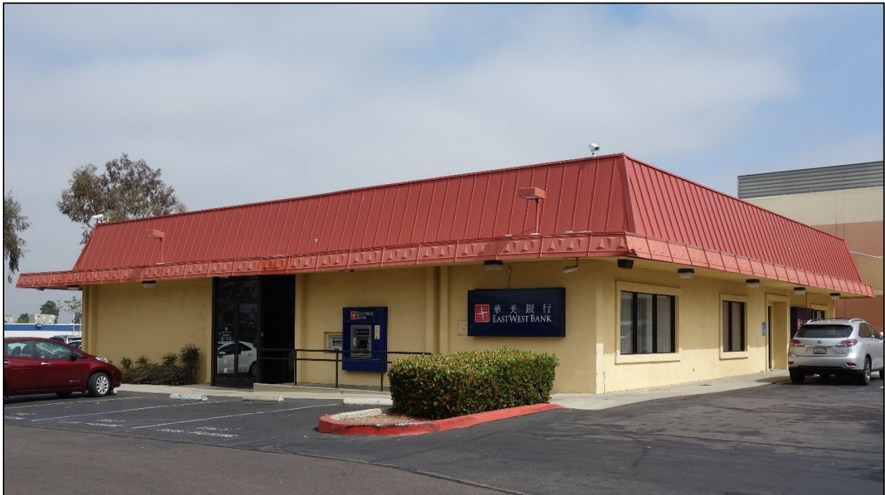
Fig. 41. The pressed metal detail on this bank at 7320 Clairemont Mesa Boulevard is one of the rare instances of decorative metal on commercial, retail, and office buildings. IS Architecture, 2018.
