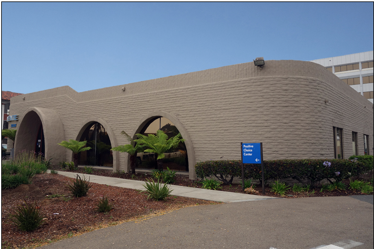
Fig. 24. A Kaiser Permanente site at 7035 Convoy Court. This building's slump block approximates the appearance of an adobe block. IS Architecture, 2018.
