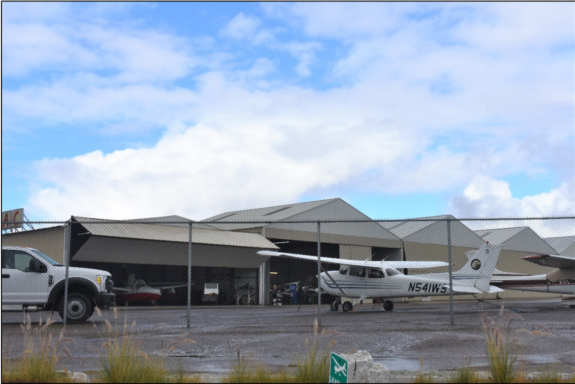
Fig. 13. Pre-engineered aviation hangars belonging to the National Air College and located at Montgomery-Gibbs Executive Airport. Notice the metal siding, flat and gabled roofs, as well as the large sliding and bi-folding hangar doors. IS Architecture, 2018.
