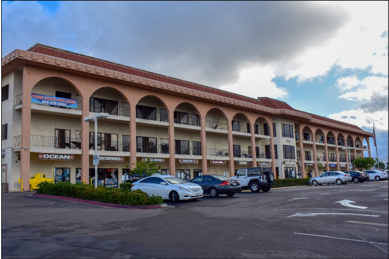
Fig. 39. The Neo-Spanish Eclectic elements of this low-rise office park building at 7710 Balboa Avenue include a red tile roof, arched colonnade, stucco façade, and red, faux tile roof. IS Architecture, 2018.
