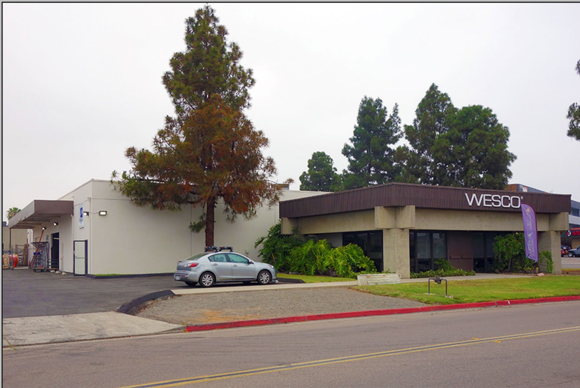
Fig. 21. The WESCO building at 7790 Convoy Court features all the character-defining features of the Office-Production type including single story massing, a styled front office attached to the warehouse space, a paved parking lot, and loading area with warehouse doors. IS Architecture, 2018.
