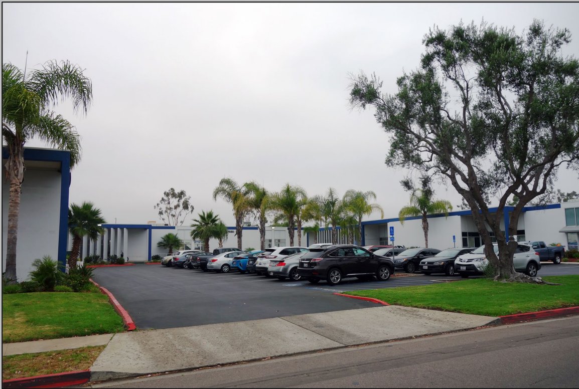
Fig. 23. Industrial park at 7701-7725 Convoy Street. This one story Industrial Park Complex features a shared parking lot, designed landscape spaces, multiple buildings with unifying details, and modern styling. IS Architecture, 2018.
