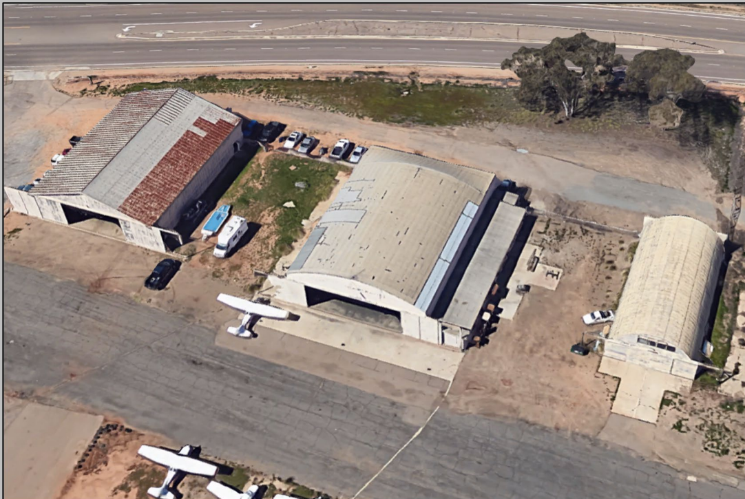
Fig. 11. These three hangars are likely the first aviation related structures in Kearny Mesa. Each display the character-defining features noted above. Google Maps, 2018.
