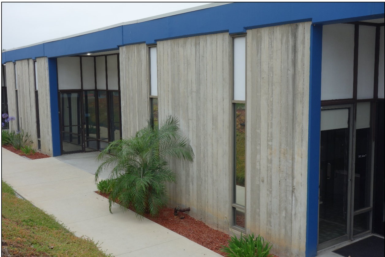
Fig. 26. Board-formed concrete is the main decorative finish on this Industrial Park Complex building at 7197 Convoy Court. IS Architecture, 2018.
