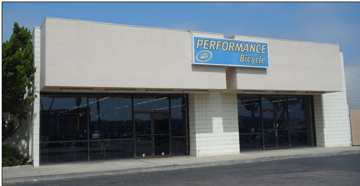
Fig. 40. This strip mall building at 7730 Ronson Road uses the short ends of the CMUs to create the appearance of square blocks. IS Architecture, 2018.
