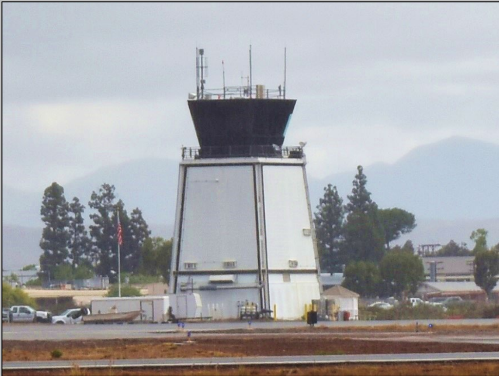
Fig. 12. The Control Tower at Montgomery-Gibbs Executive Airport. IS Architecture, 2018.
