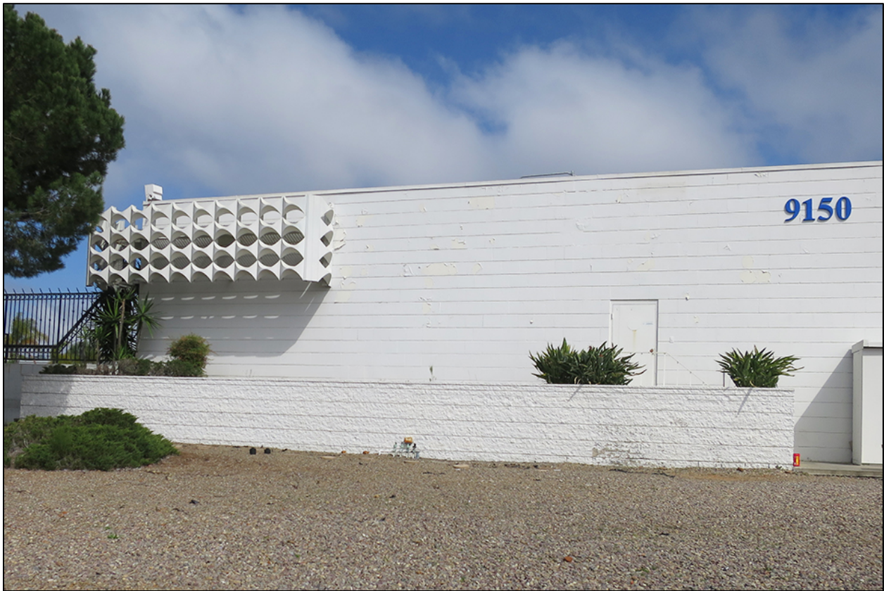
Fig. 27. Decorative pierced metal wraps around the corner of this CMU industrial building at 9150 Balboa Avenue. IS Architecture, 2018.
