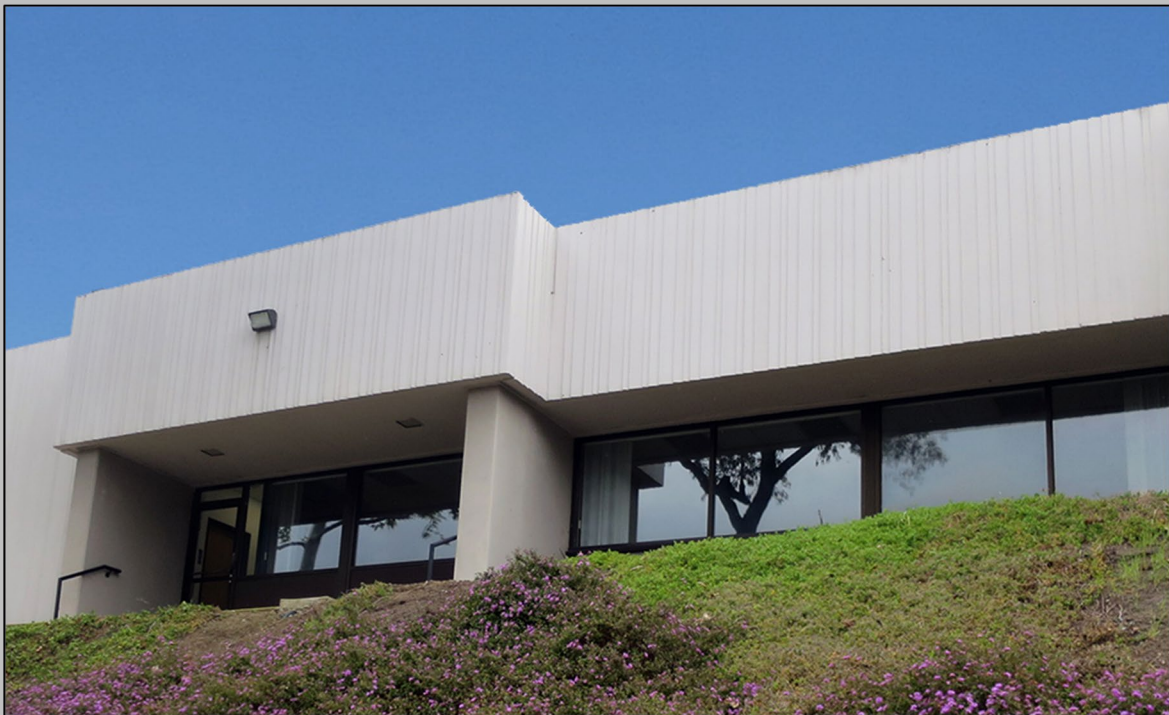
Fig. 38. This office park building at 9465 Farnham Street is one of a complex of three low-rise office buildings with designed landscaping beds around each building and along the street frontages. A continuous, paved parking lot connects the buildings to each other, and the board formed concrete detailing is a distinctive Modern design element that unites the buildings. IS Architecture, 2018.
