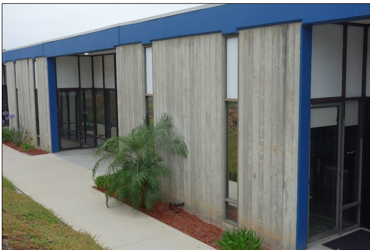
Fig. 23. Board-formed concrete is the main decorative finish on this Industrial Park Complex building at 7197 Convoy Court. IS Architecture, 2018.
