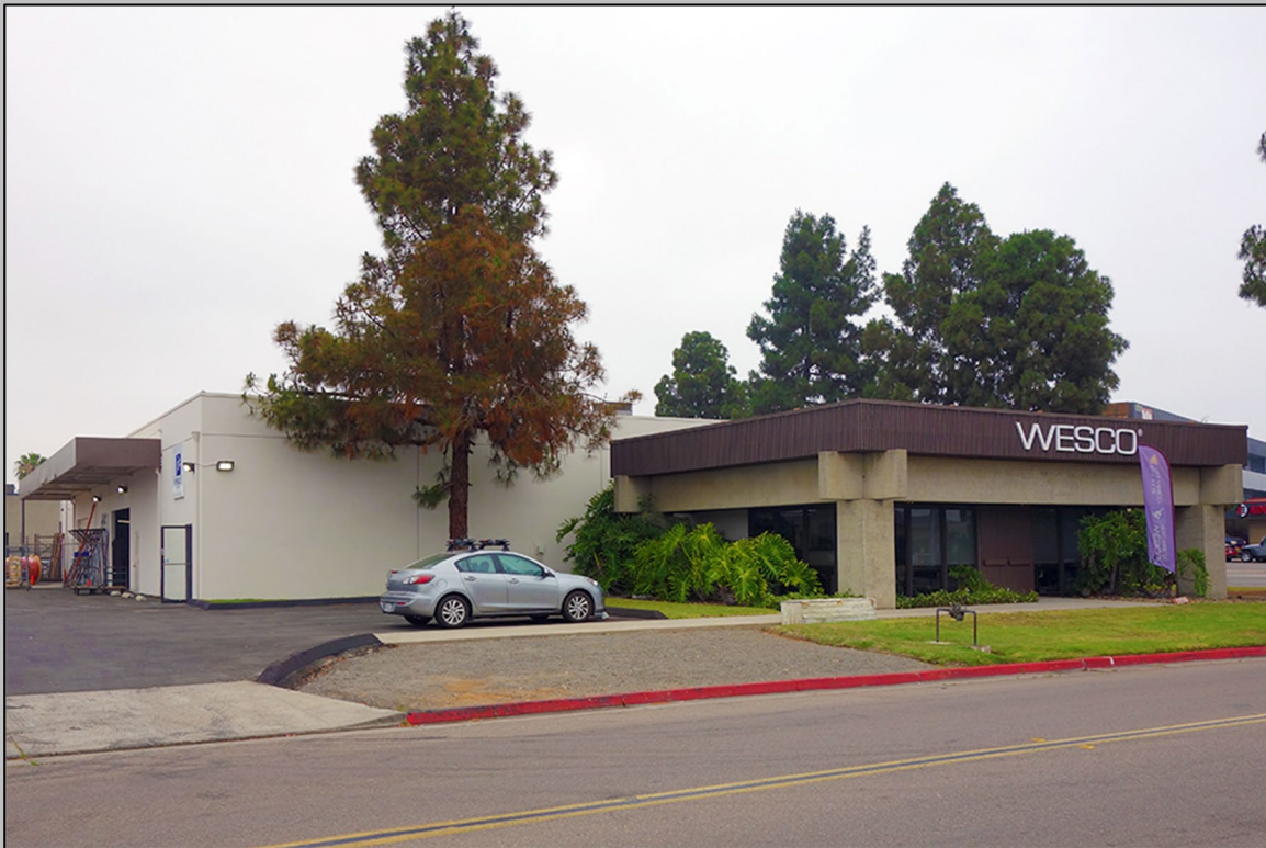
Fig. 18. The WESCO building at 7790 Convoy Court features all the character-defining features of the Office-Production type including single story massing, a styled front office attached to the warehouse space, a paved parking lot, and loading area with warehouse doors. IS Architecture, 2018.
