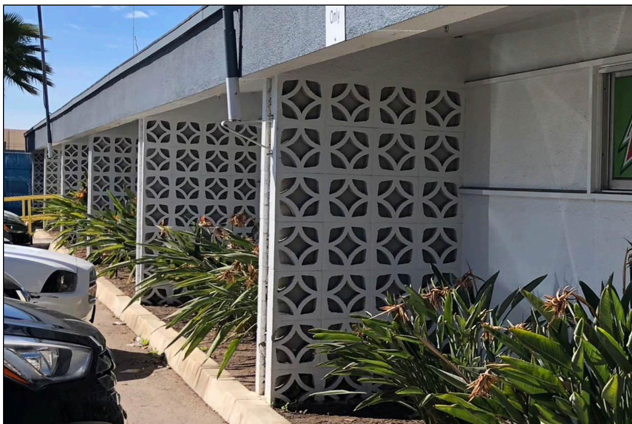
Fig. 25. Decorative pierced block screens on the Pepsi Cola bottling plant at 7995 Armour Street. IS Architecture, 2018.
