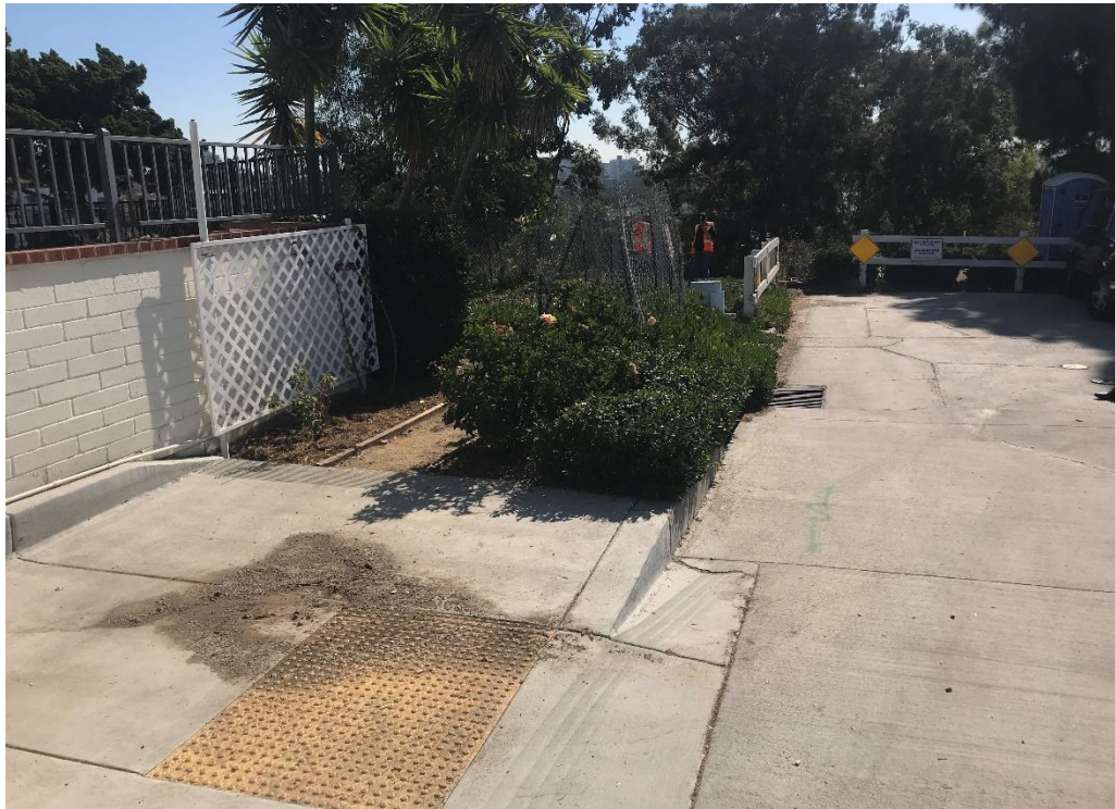
Photo 6. Southeast-facing view of storm drain inlet location.
