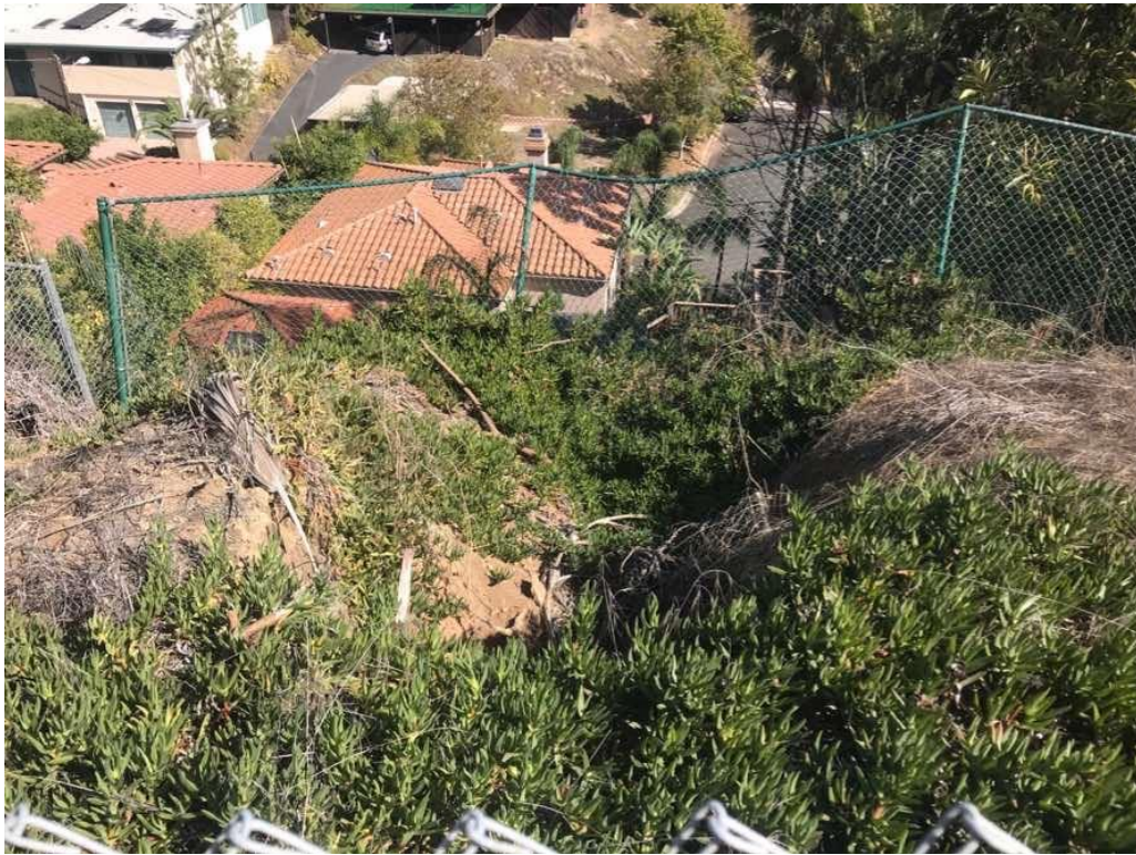
Photo 7. East-facing view of failed storm drain pipe at sinkhole location.
