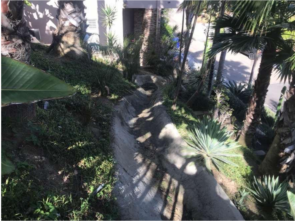
Photo 9. North-facing view of existing concrete brow ditch.
