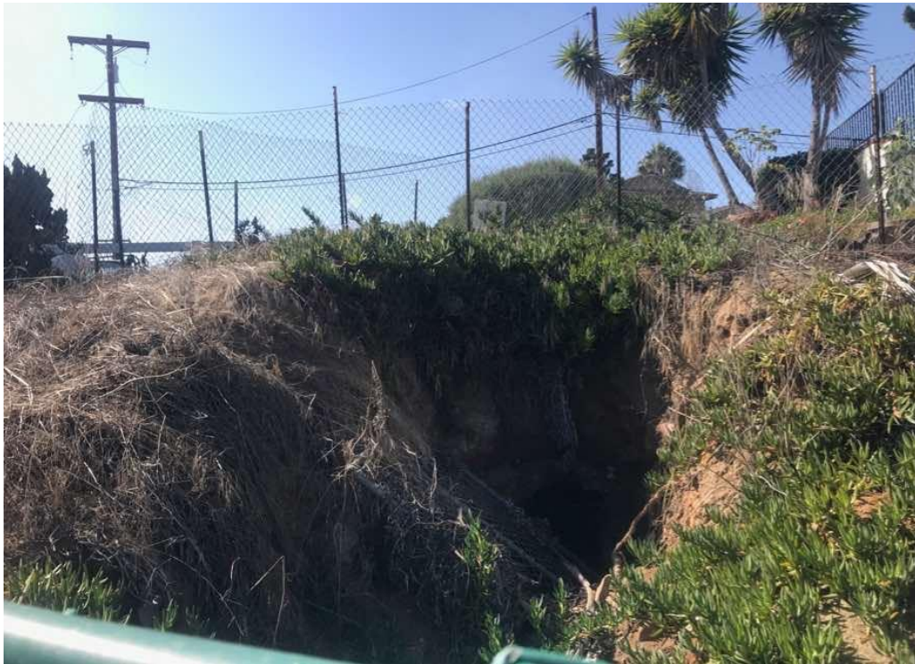
Photo 8. West-facing view of failed storm drain pipe at sinkhole location.
