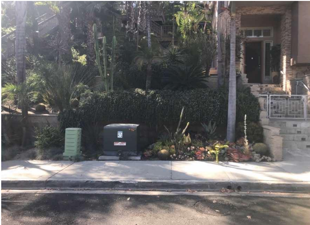
Photo 4. Southwest-facing view of storm drain cleanout location.
