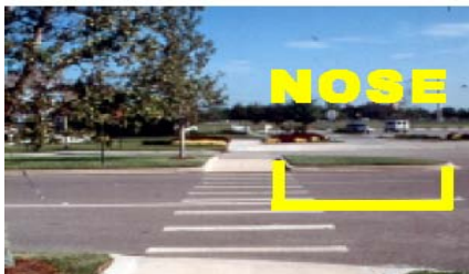
In the photo above, note that the sidewalk is set back from the end of the median by a considerable amount. This median nose provides separation between those crossing the street and turning vehicles.
