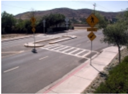
The principle of offsetting the pathway in a refuge island was developed to prompt pedestrians to change their direction and look at oncoming traffic. An angled path, as shown in the above photo, or a linear path as shown in the photo below, will both achieve this goal. The path in the bottom photo is fenced to prevent shortcutting.
