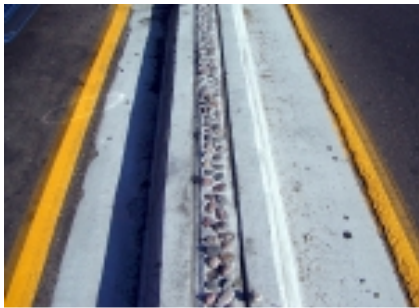
If the roadway is properly sloped, these gutters are unnecessary. Make the median itself wider instead.
