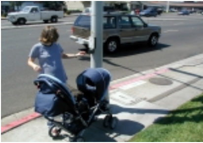
The location of pedestrian push buttons and the design of ramps along Balboa Avenue often inconvenience walkers.
