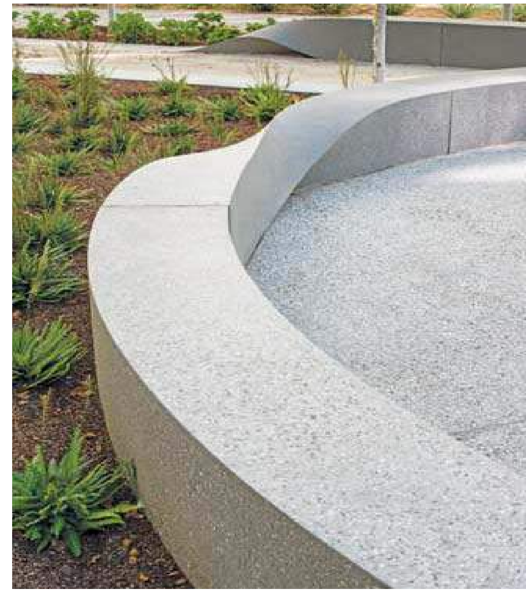
CONCRETE DIVERTING WALL
