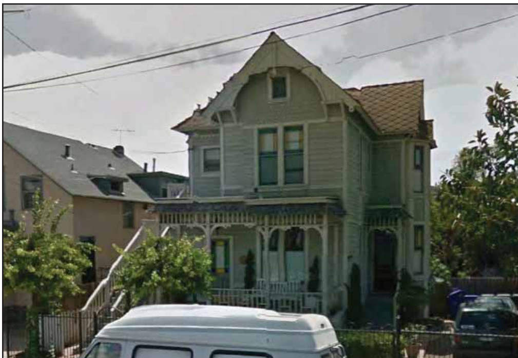
Figure 5.15-6: Traditional single-family home in Southeastern San Diego
