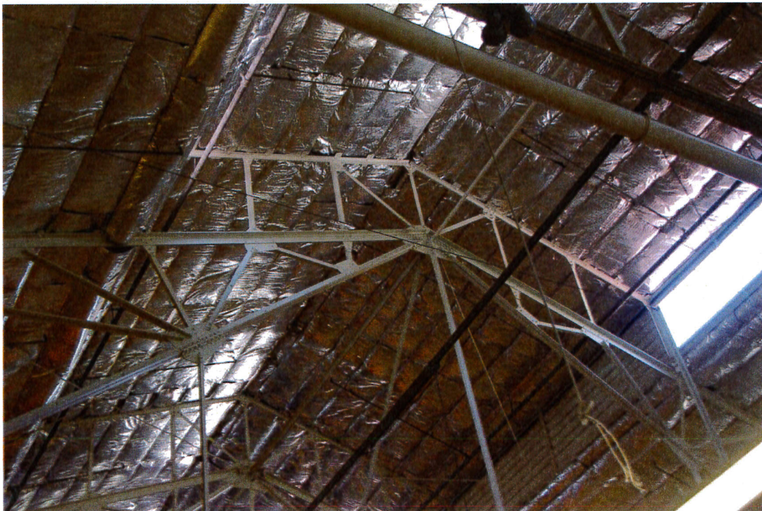
Photo 4: 372 Fourth Avenue – roof trusses.
