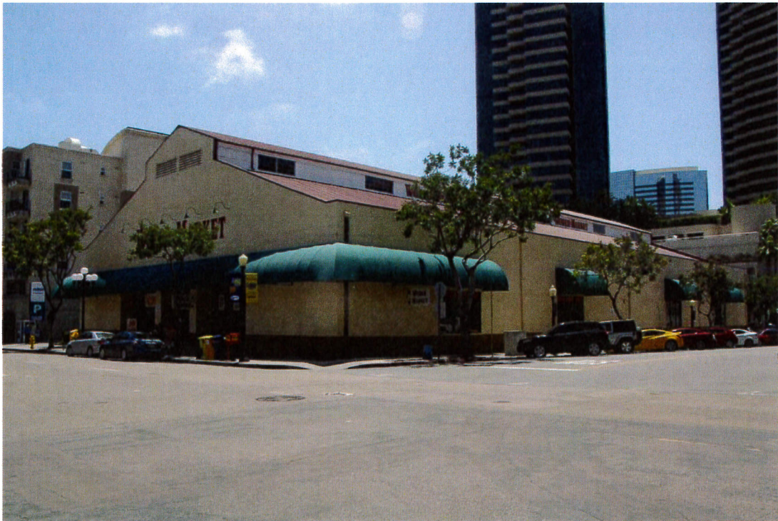
Photo 1: 372 Fourth Avenue with new storefront openings, roof and awnings.
