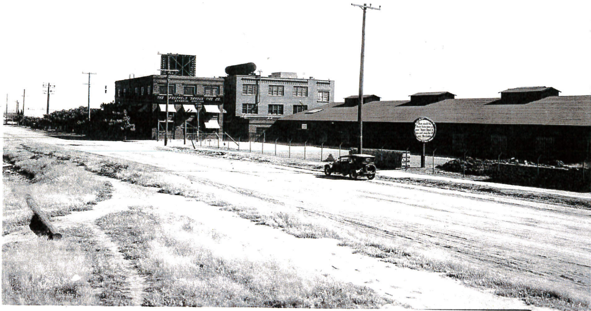
S-432 SENSOR SPRECKELS SAVAGE TIRE CO. Savage Tire Co. on 26 th Street. Brick and wood construction on exterior. Note monitor form on roof.
