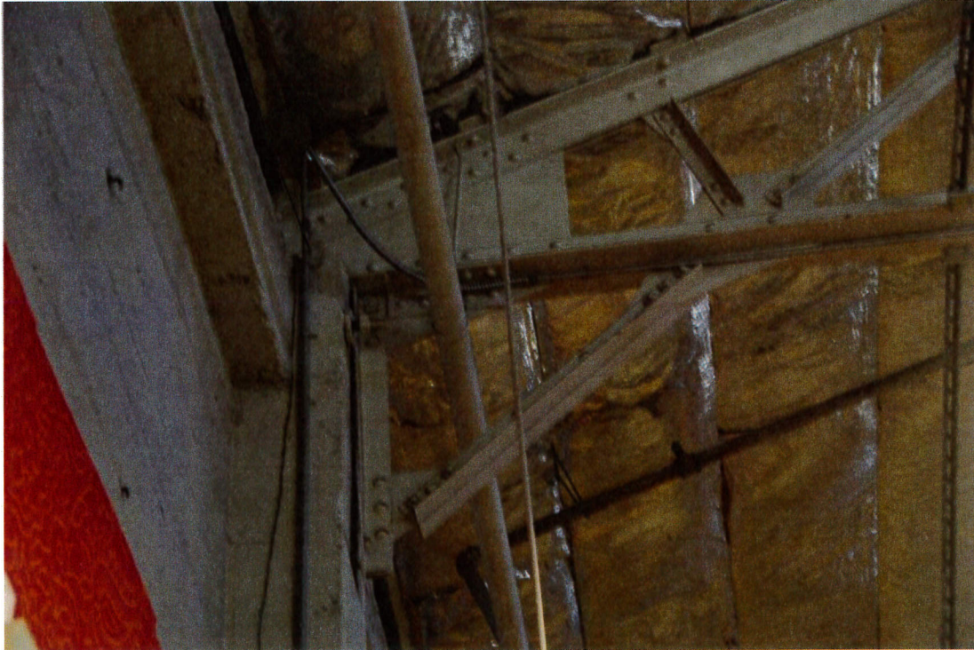
Photo 3: 372 Fourth Avenue – roof trusses.
