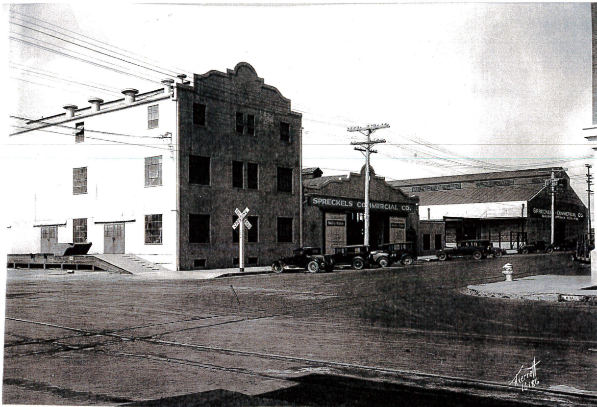
Looking North from "K" Street. Older warehouse buildings constructed in wood with "Mission Revival" Parapet at street elevation. The spreckles Warehouse exhibits strong building form without direct historical reference. There is no "front" or "back", evoking one of the modernism tenants: form follows function.
