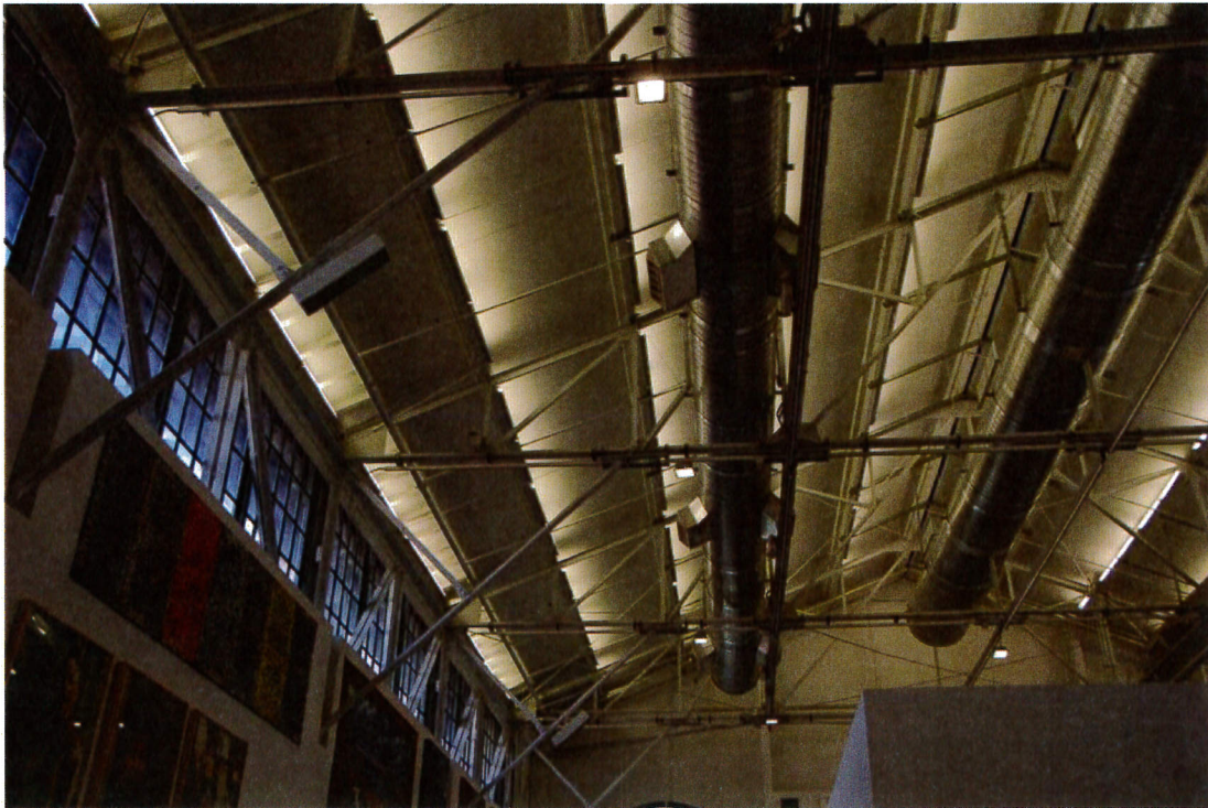
Photo 6: MoMA Roof Trusses
