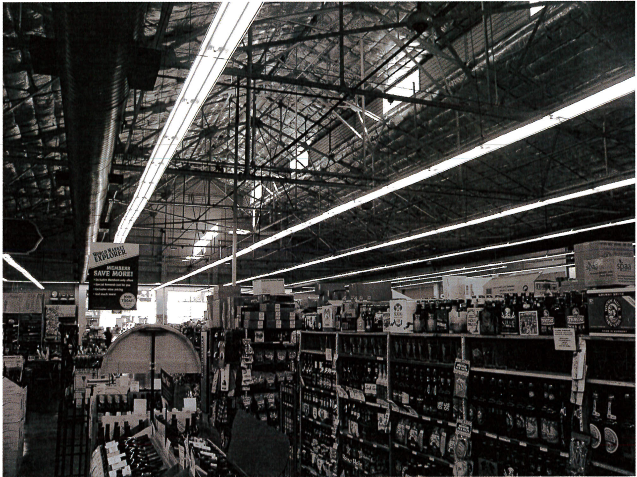
Interior photograph showing steel roof truss spanning one hundred feet at 20'-0" on center spacing. Note end wall at gable is constructed of poured concrete.
