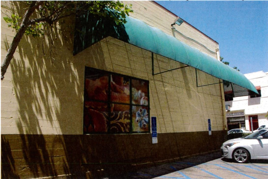
Photo 2: 372 Fourth Avenue – board formed concrete, removed loading dock, modified openings and new awnings.
