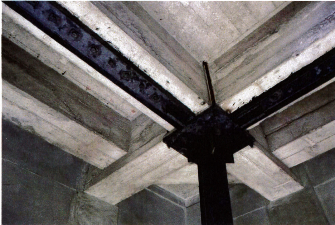
Photo 8: Museum of Man – board formed concrete and steel bracing at Tower.
