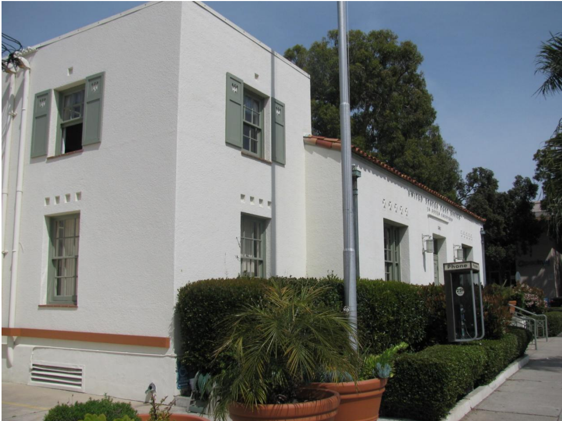
West end, south elevation, March 2013
