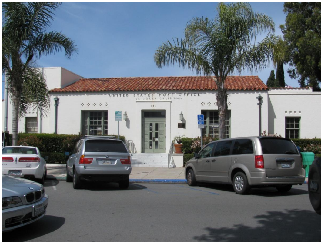
South elevation, March 2013
