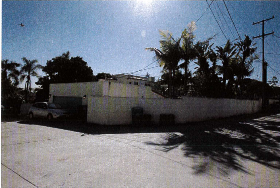
Photo 1: View from the alley showing the second floor addition on the tertiary facade.
