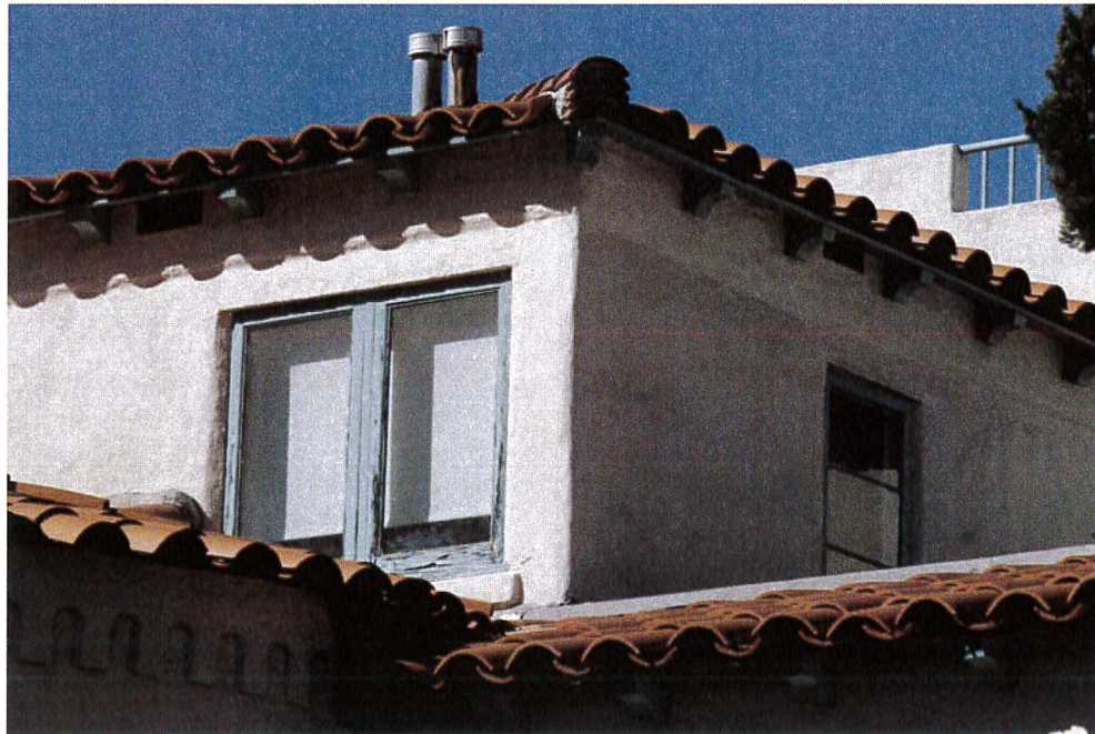
Photo 2: View of second floor from the primary façade with the addition visible beyond.
