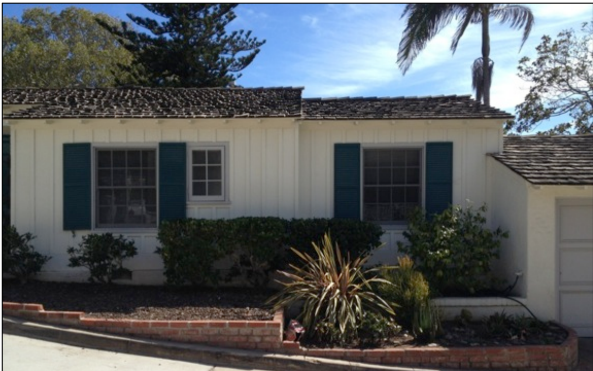
North Elevation-West End
