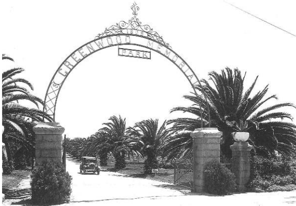
Figure 12. Decorative gate at Greenwood Memorial Park, 1920. (San Diego History Center Photo Archive, #2357-D)
