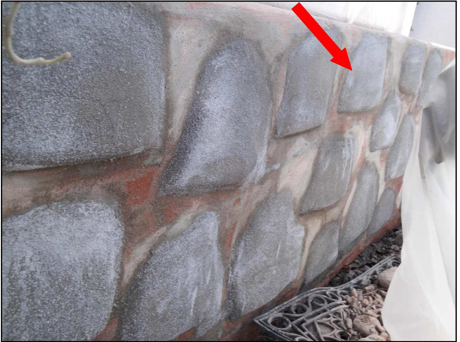
Figure 2 3127 McKinley Street Front façade during restoration. Raised hand troweled finish shown with red arrow. Photo below by Kiley Wallace, February 2015
