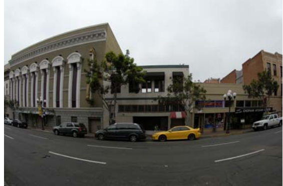
C. 6TH AVE. VIEW FACING WEST
