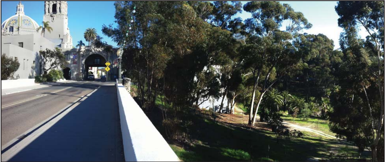
View of Cabrillo Bridge without Centennial Bridge
