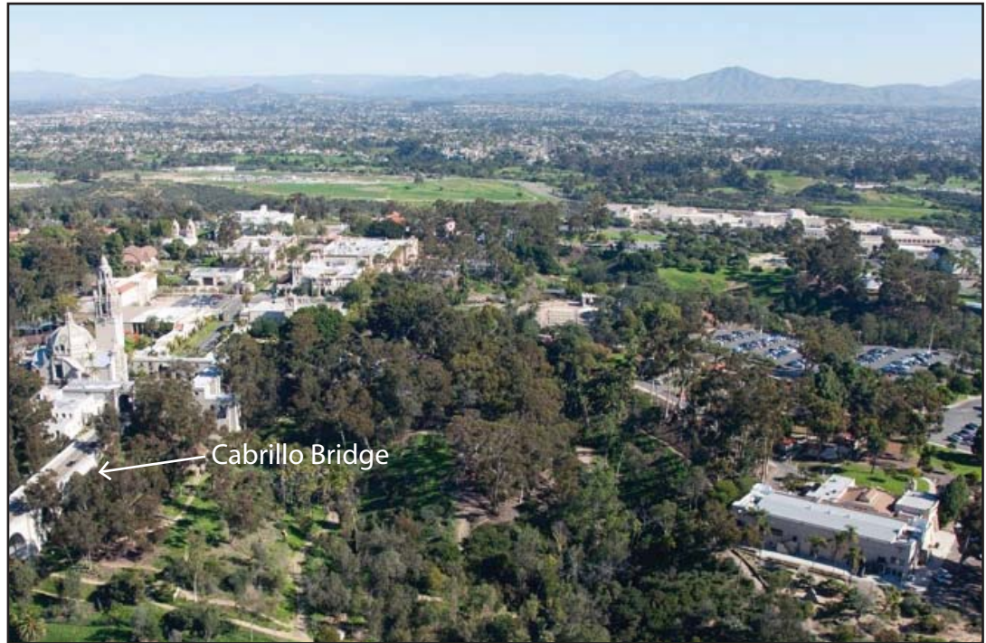
View of Cabrillo Bridge without Centennial Bridge
