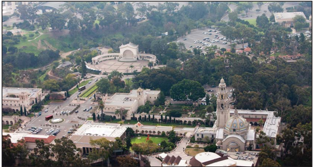
Existing Parking Lot from North
