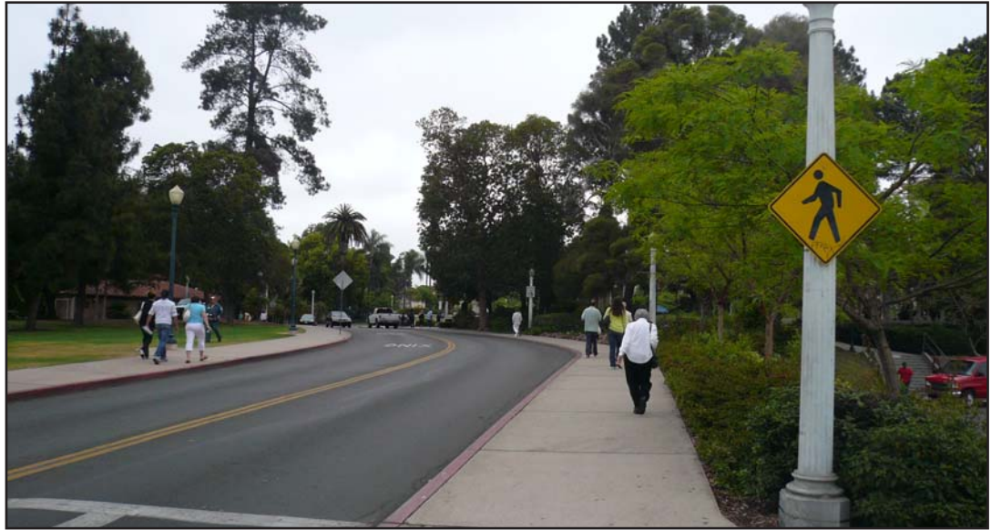
Existing Pan American Road East
