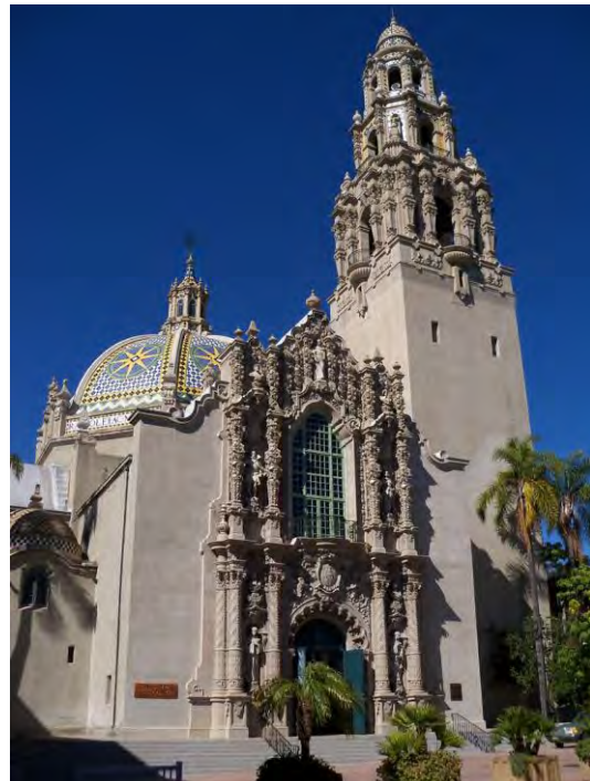
Figure 34. California Building Source: Christopher VerPlanck
