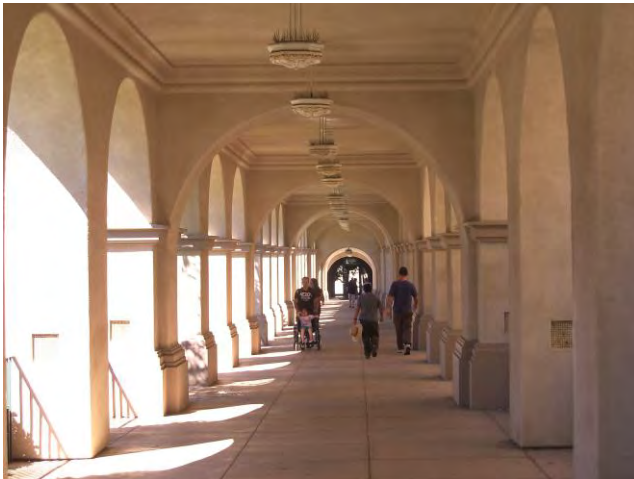
Figure 39. West Arcade Source: Christopher VerPlanck
