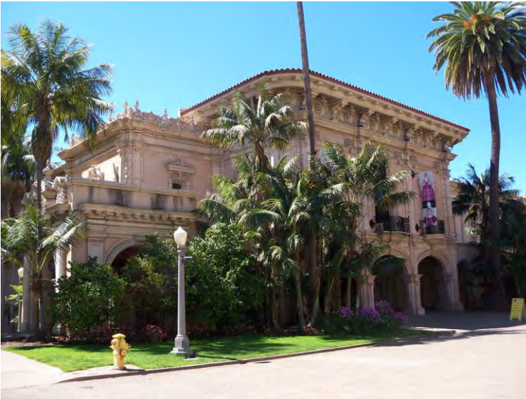
Figure 49. Casa de Balboa, view toward southeast Source: Christopher VerPlanck
