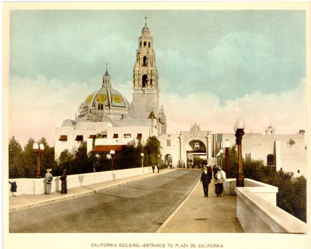
Figure 18. California Quadrangle from Cabrillo Bridge, looking east Source: Collection of David Marshall, AIA
