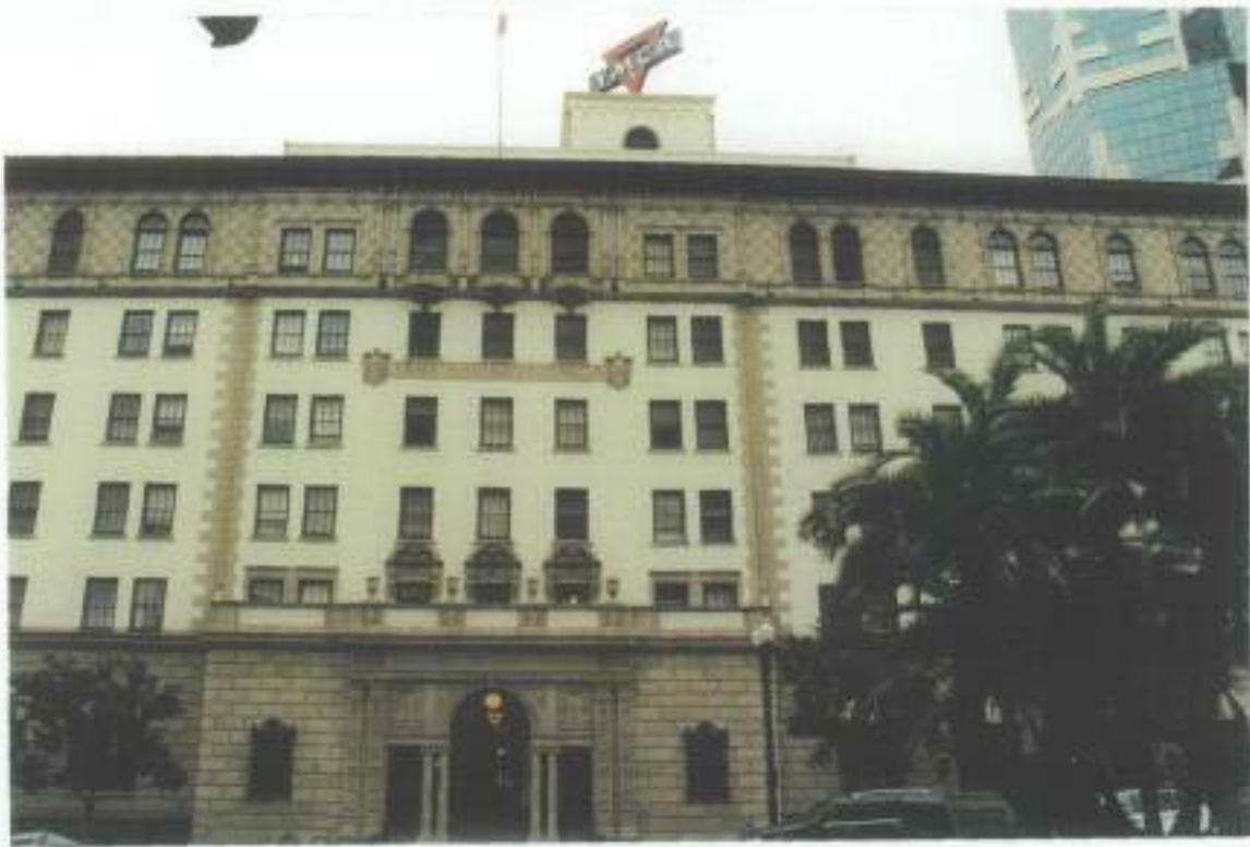
View to North of South Facade and Tower
