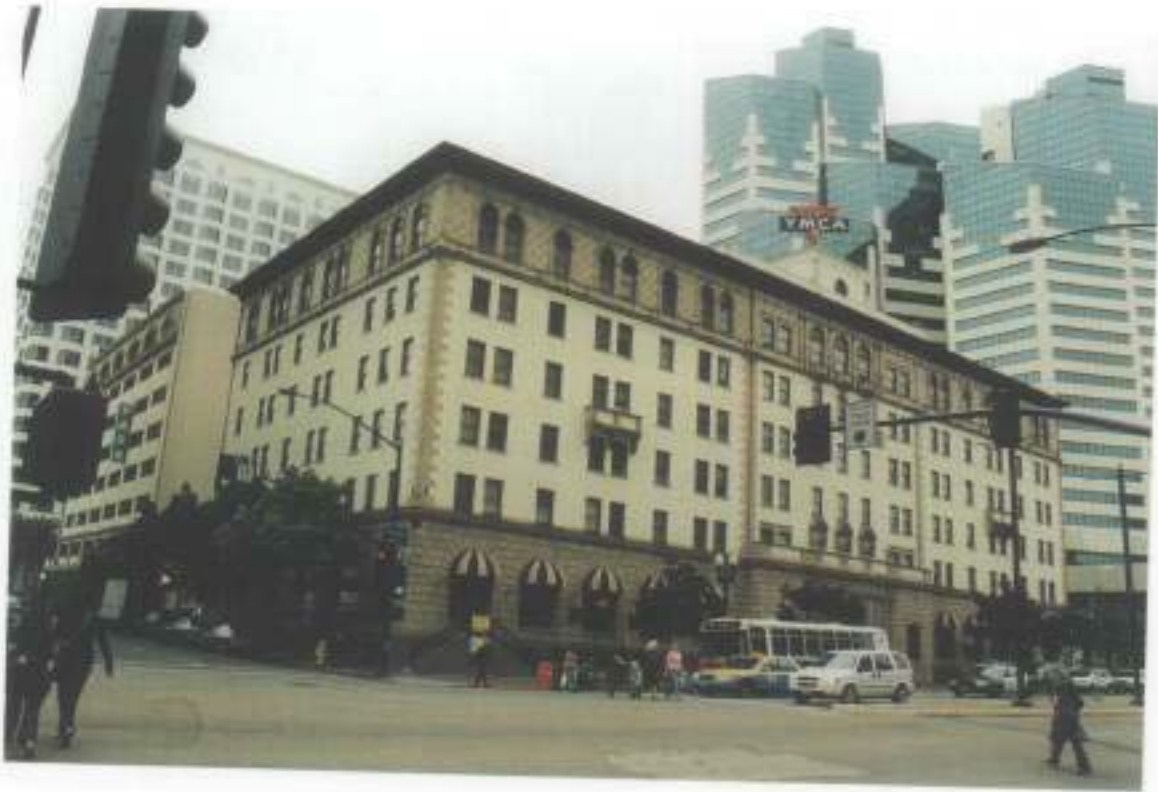
View to North East of South and West Facades
