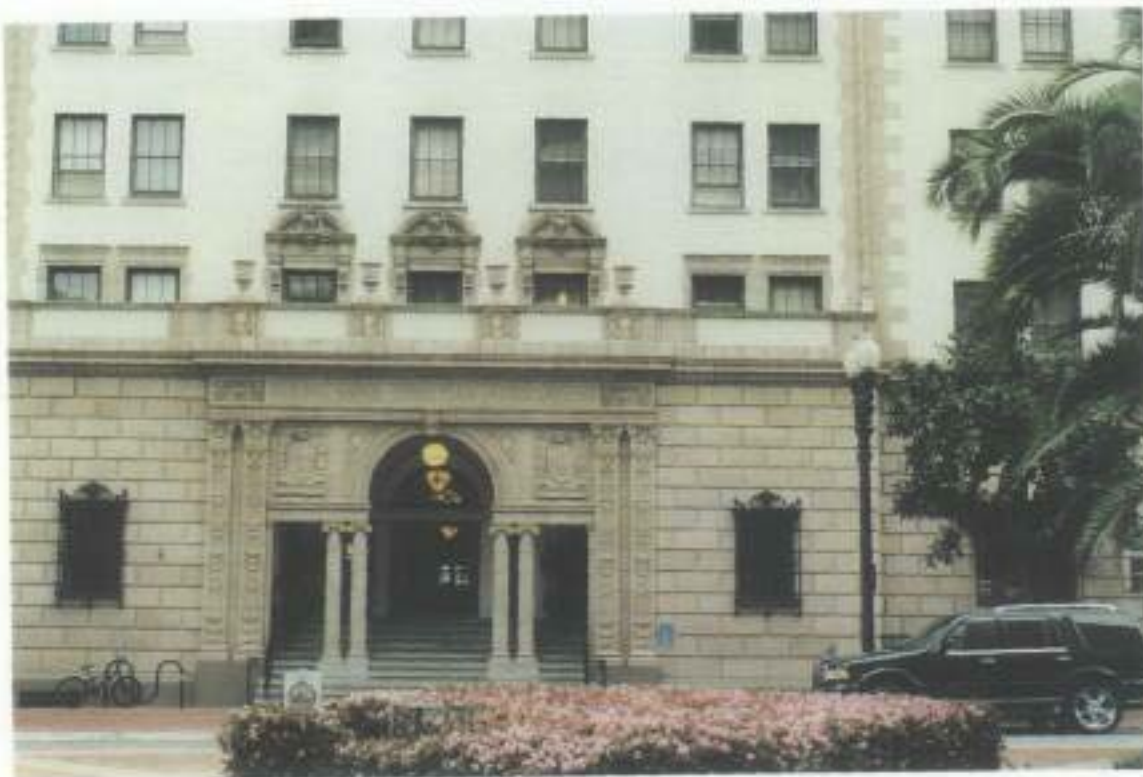
View to North of Central Pavilion on South Facade
