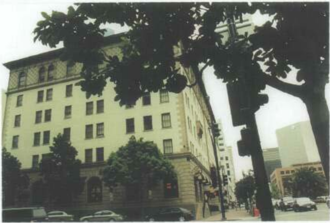
View to East of West Facade
