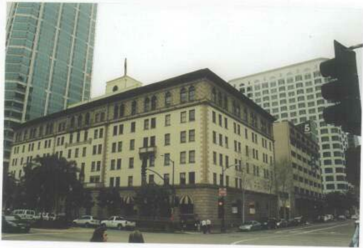
View to North West of South East Facade
