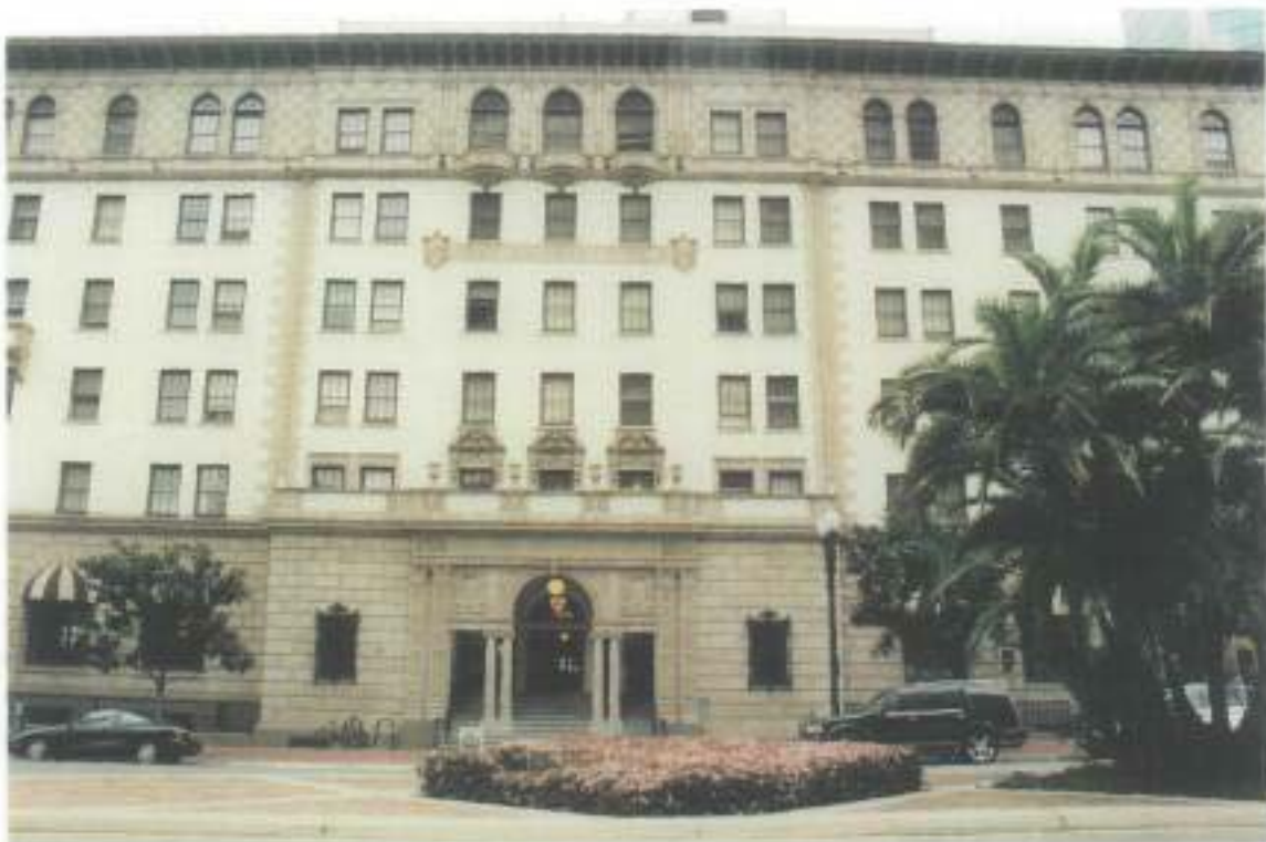
View to North of South Facade
