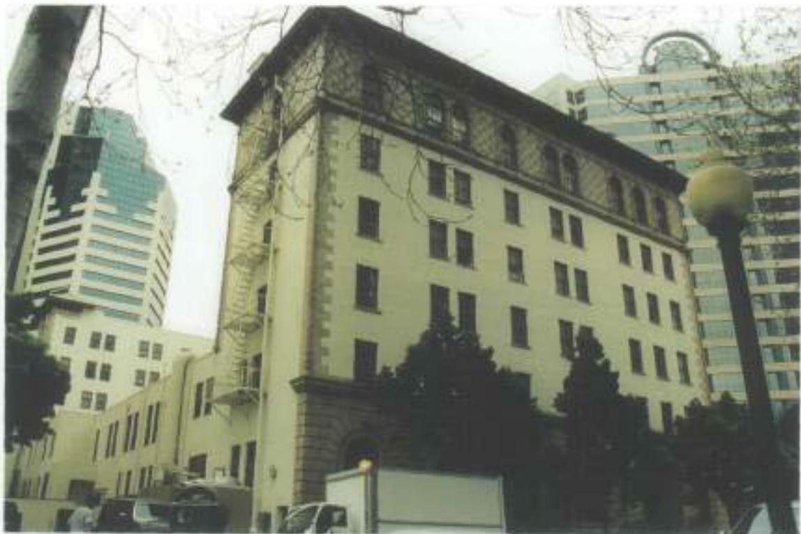
View to South East of West Facade
