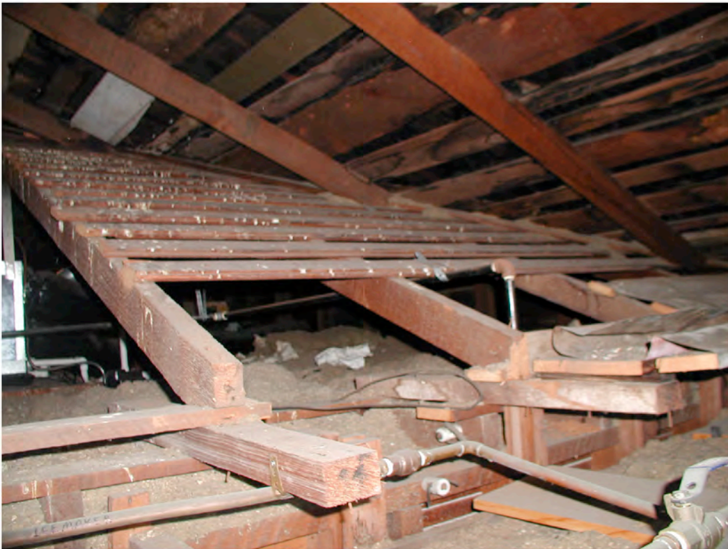
#2 PHOTO: View of attic showing roof framing at west gable addition 1909-1921. Note skip sheathing of main roof with new cross gable framing above. All lumber dimensions are the same.
