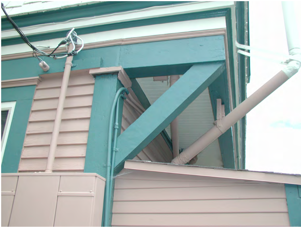
#5 PHOTO: Non-original corner knee brace at south -bump out- addition.
