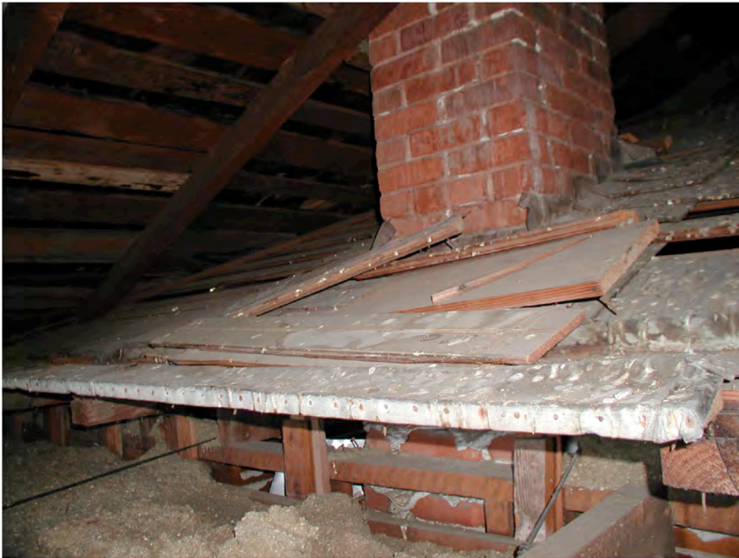
#1 PHOTO: View of attic showing roof framing at the west gable addition 1909-1921. Note the flashing left in place, lower ceiling joists above original porch.
