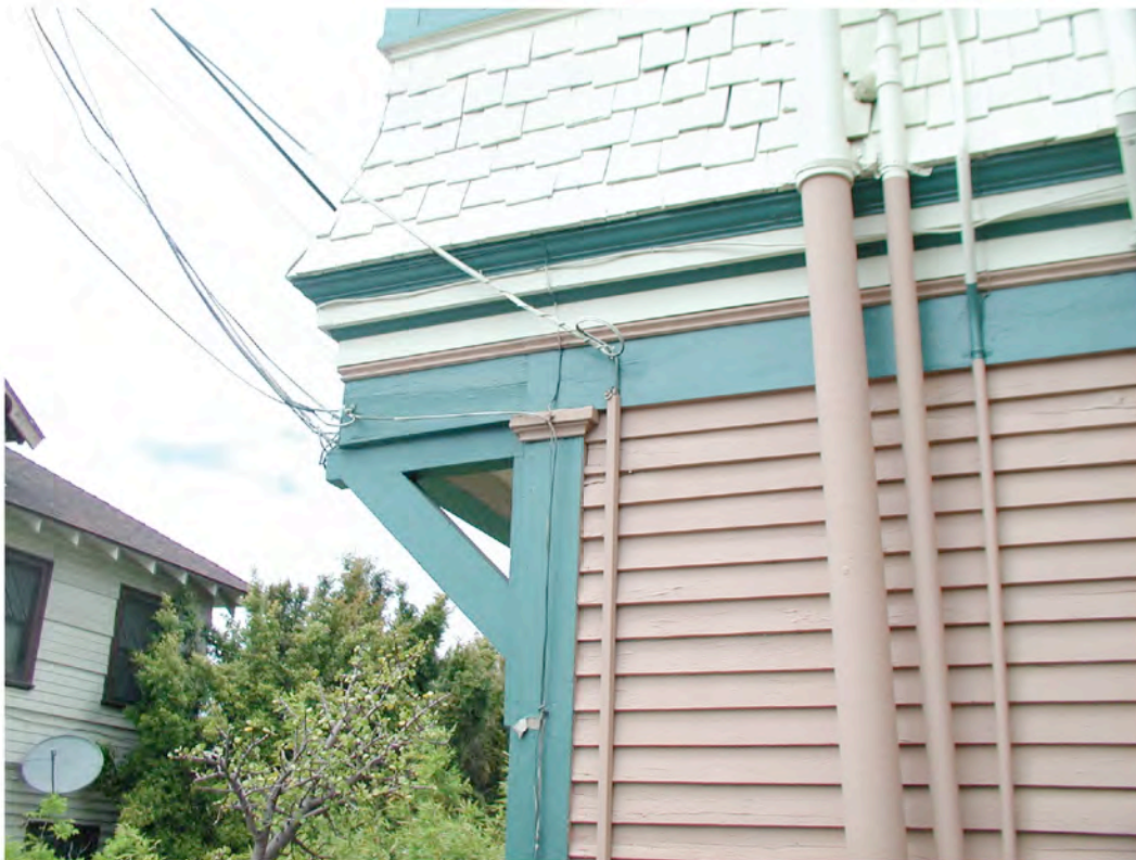
#4 PHOTO:Original corner knee brace at west-bumpout- addition.
