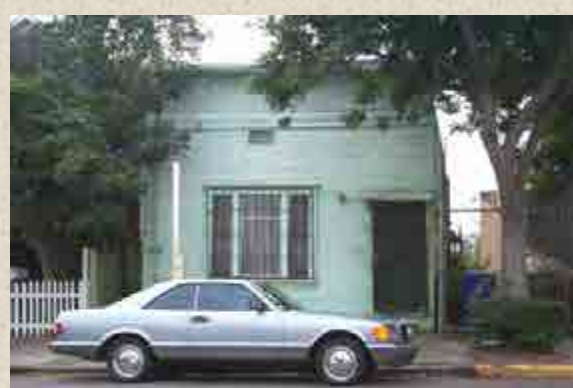
20. 1451-1453 F Street (EV) Residence 1889-1890
