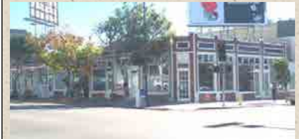
17. 801-821 F Street (EV) Rossi Business Block 1924
