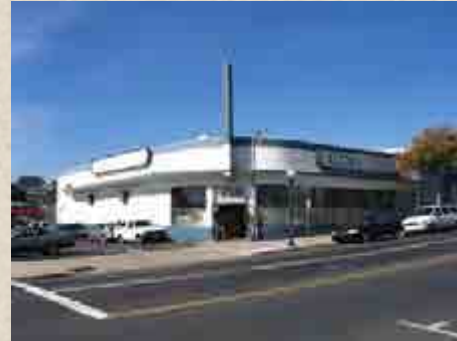
69. 716 16 th Street (EV) Todd's Market c. 1947
