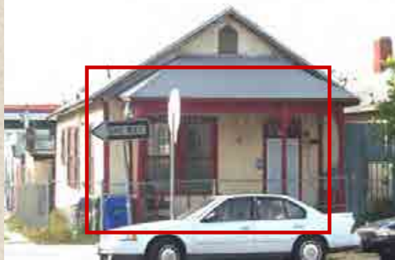
77. 508 17 th Street (EV) Falkenstein House c. 1887
