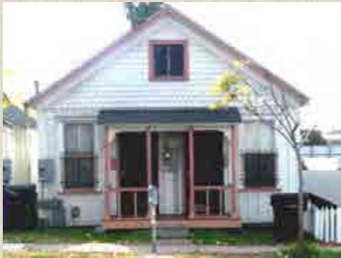
5. 1321 C Street (EV) Residence c.1887
