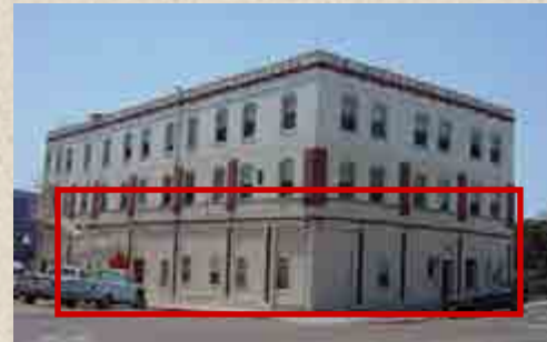
29. 1335 J Street (B) Hotel Salem/Workman Hotel 1912
