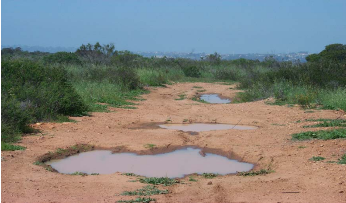
Shaw Texas Road ruts 8, 9, and 25 (near to far) looking northwest
