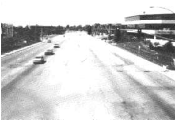
The wider the street the greater the need for landscaped medians to break the vast expanses of asphalt.
