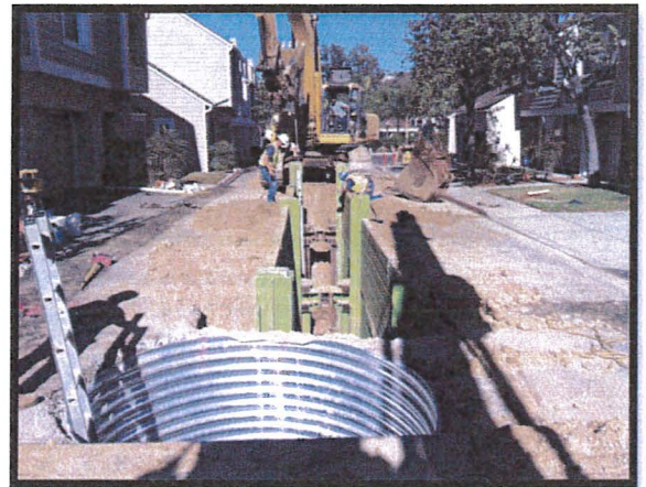
Open trench construction of sewer main and manhole.
