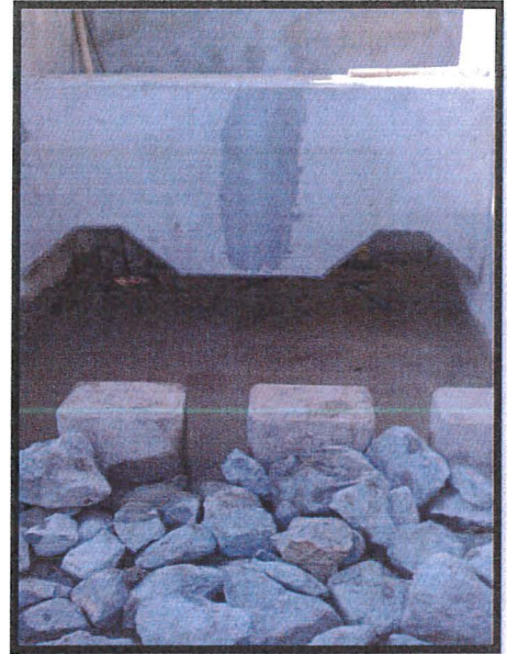
Concrete energy dissipater apron and baffle blocks.
