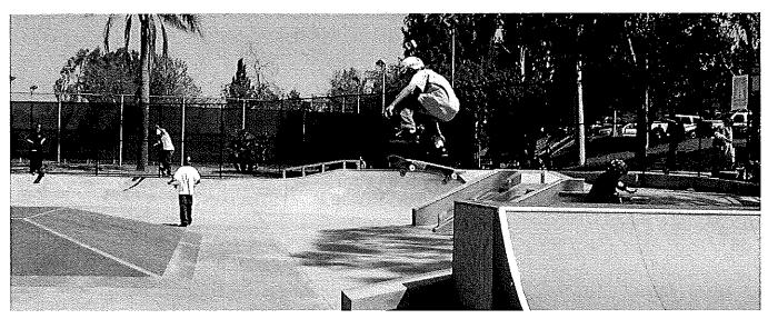
The La Mesa Skate Park street course consists of wood structures with polymer decking, concrete transitions, concrete stairs, grind rails and a 2,000-square-foot concrete bowl with both five-foot and seven-foot depths. The park includes staging area including a temporary building, vending machines, portable restrooms, picnic tables, benches and lockers.
