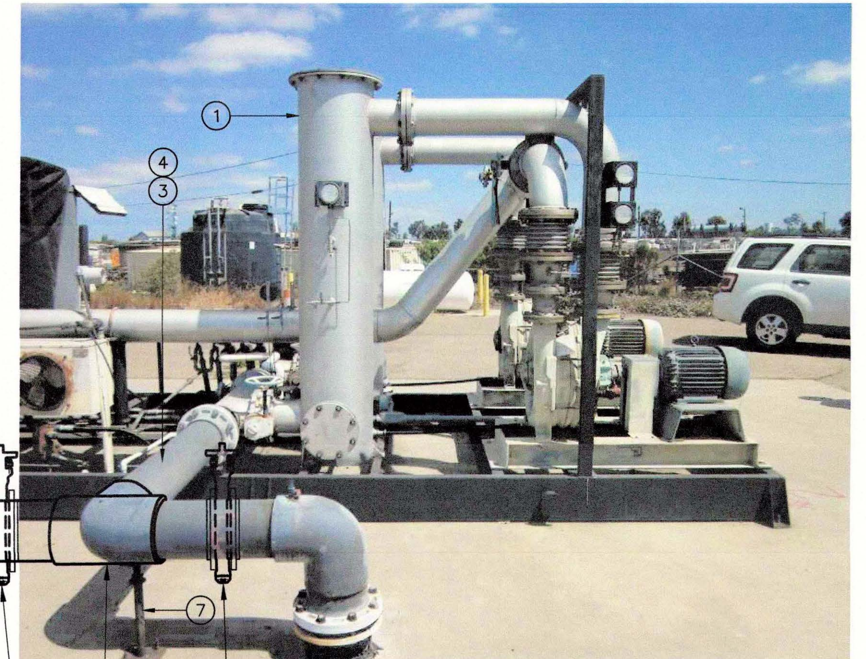
HOLY SPIRIT LFG FLARE CONNECTION DETAIL
