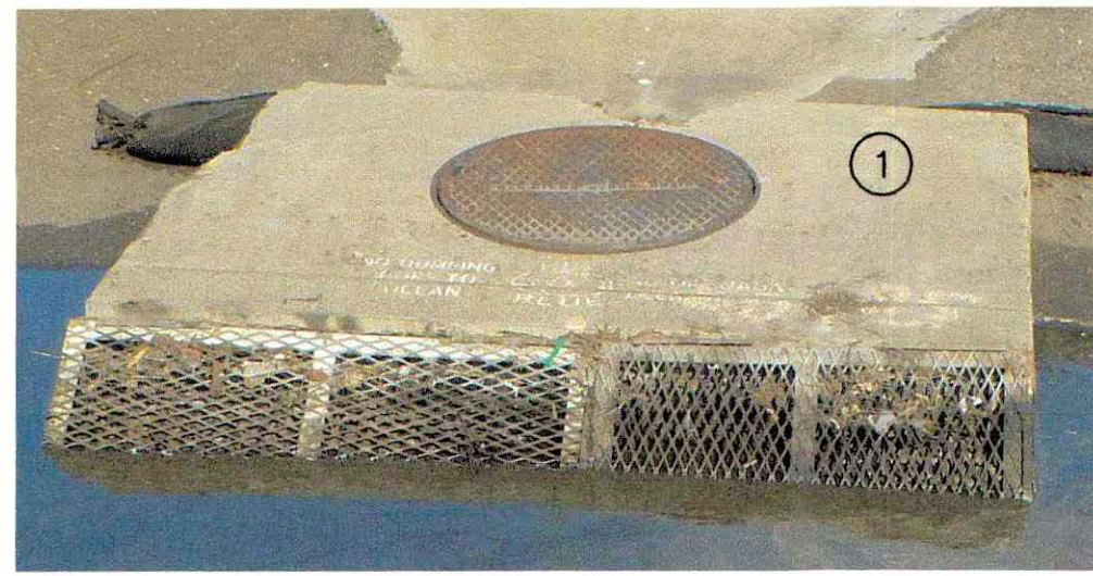
EXISTING DRAINAGE INLET
