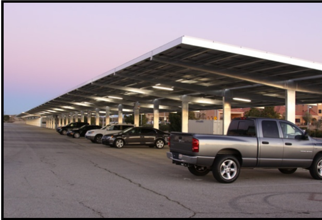
Figure 4.3-1. Typical T-Framed Solar Shade Canopy
