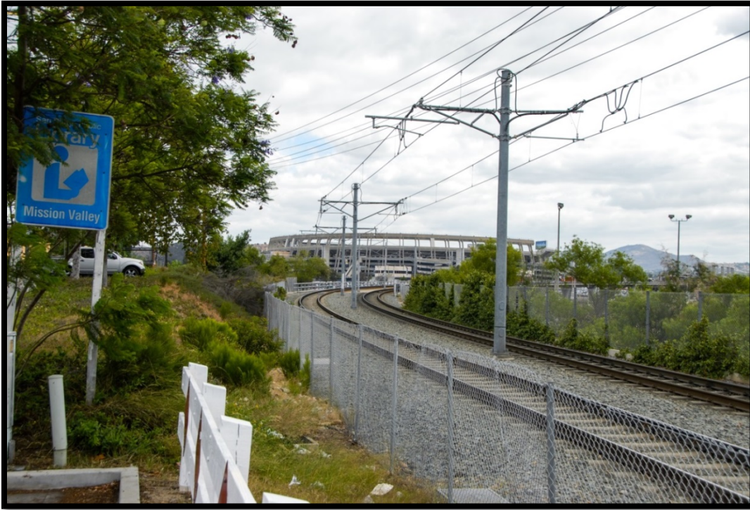
Figure 4.15-9 View 7—Eastward View of Existing Project Site from MTS Fenton Station
