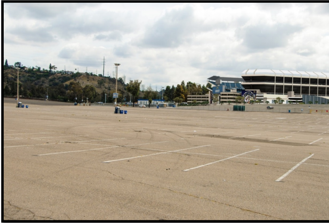
Figure 4.15-26 View 12—Northeastward View of Project from Western Parking Lot
