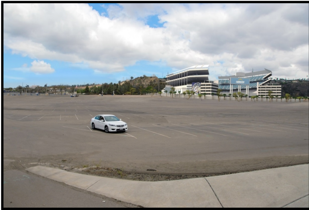
Figure 4.15-24 View 10—Northwestward View of Project from Parking Lot Corner
