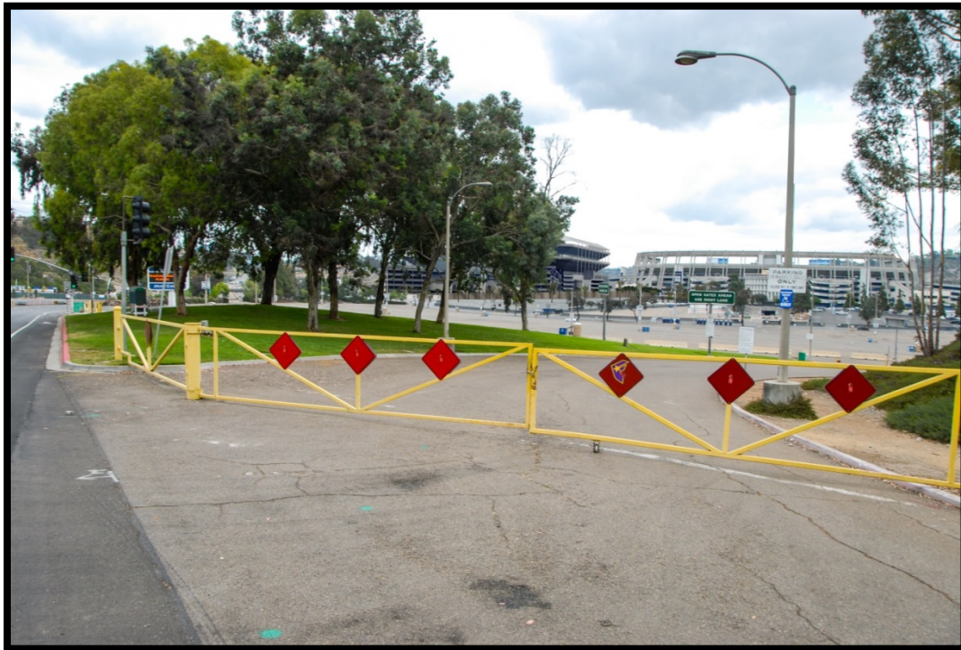
Figure 4.15-30 View 8—Eastward View of Project during Construction Phase from Friars Road
