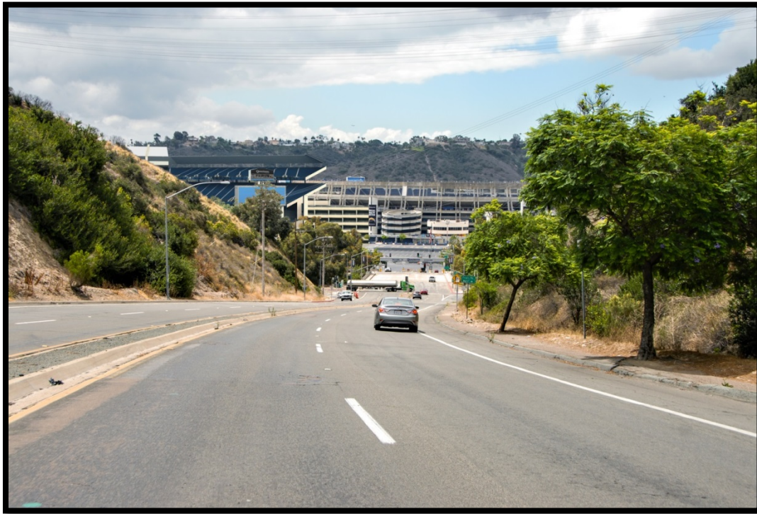
Figure 4.15-27 View 1—Southward View of Project during Construction Phase from Mission Village Drive
