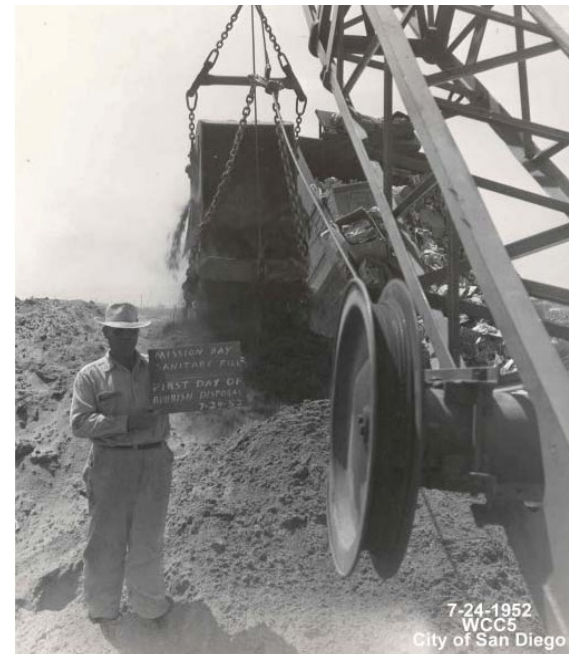
First Day of Rubbish Disposal at Mission Bay Sanitary Fill Site Source: 7-24-52 WCC3 City of San Diego
