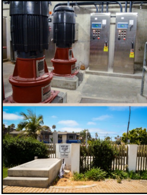
Interior and exterior views
