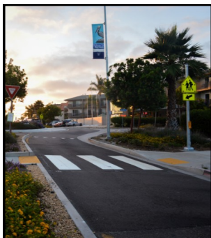
New crosswalk at Colima
