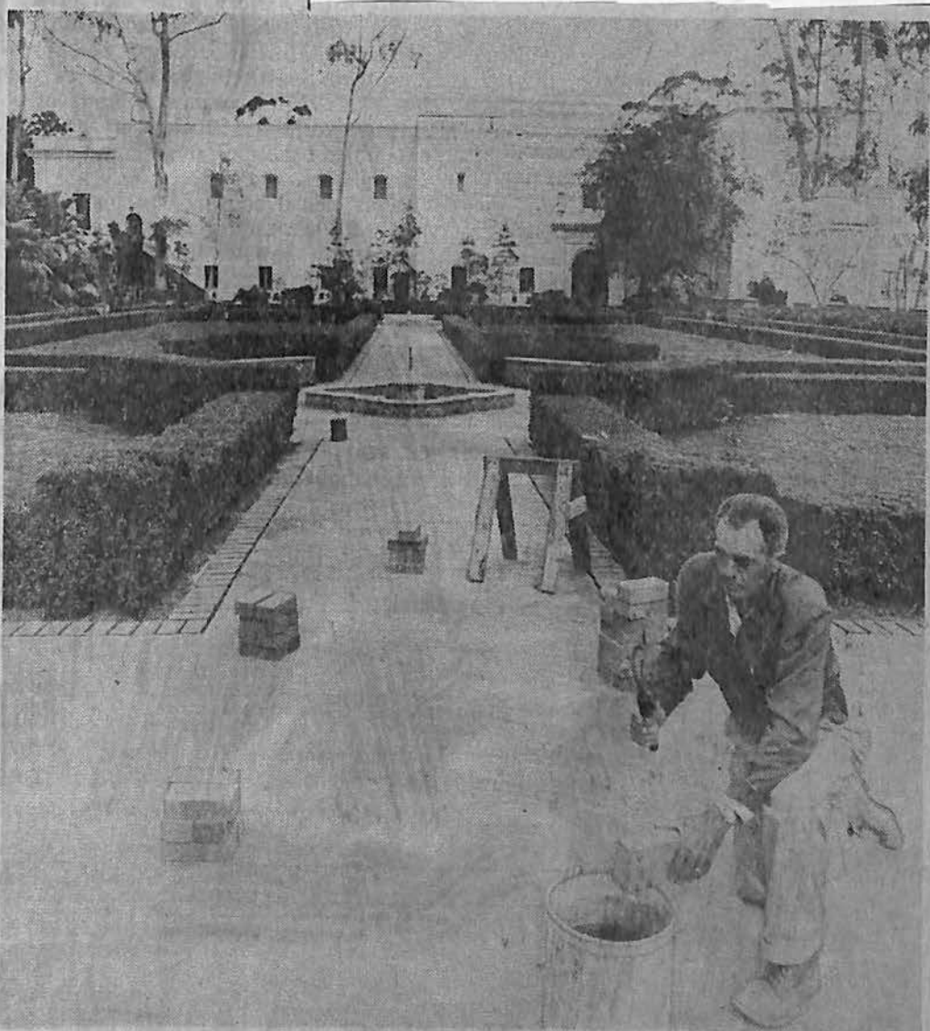
Custodian W. W. Pfahler applies finishing touches to refurbishing of
