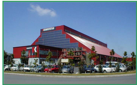
Thermoselect Facility Chiba, Japan
