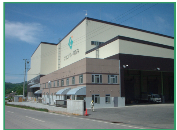
Plasma Gasification Facility Utashinai, Japan
