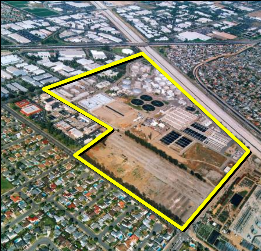
Reclamation Plant No. 1
