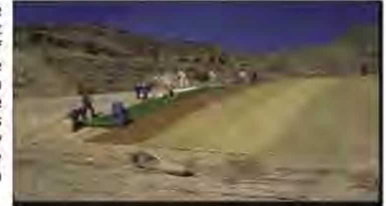
Erosion control blankets (ECBs) can be used on steep slopes, in areas of concentrated flow and around the foundations of structures to prevent soil loss.
