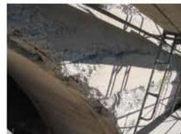
Saw cut concrete area to a rectangular shape and chip to board form
