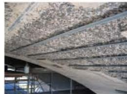
Concrete is mixed to resemble color and texture and placed on patch area to complete work as shown on the far right photo
