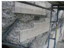
Steel is then pinned and rewired just before patching
