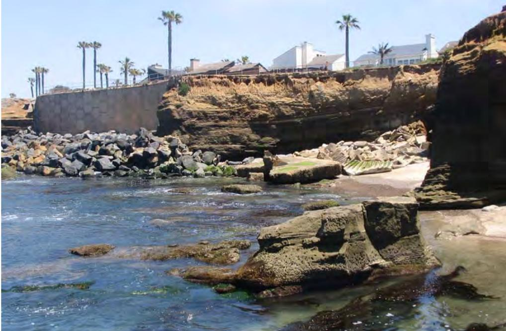
PH25/26: (Spalding Point) This arch fell about 10 years ago. In 1915 there was a seawall and viewing platform. This collapsed because the seawall failed (Dedi suspects that this is indirect erosion caused by the seawall/shore protection scouring around it).
