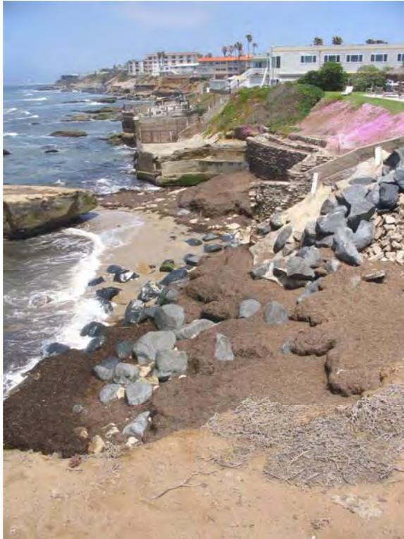
PH29: This shows 'unnatural' erosion caused by failing and settling rubble.
