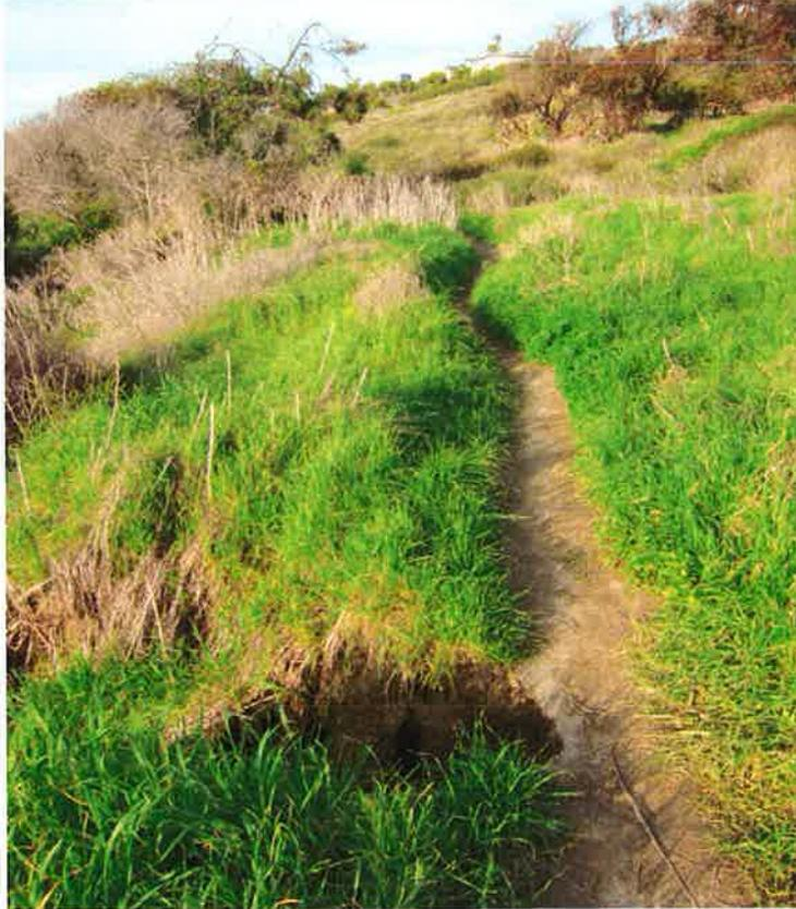
**Figure 12A.** Runoff from the 18" pipe is undercutting this trail that is being considered as a secondary trail for the Park, and has caused a significant collapse of the trail and the slope adjacent to it.
