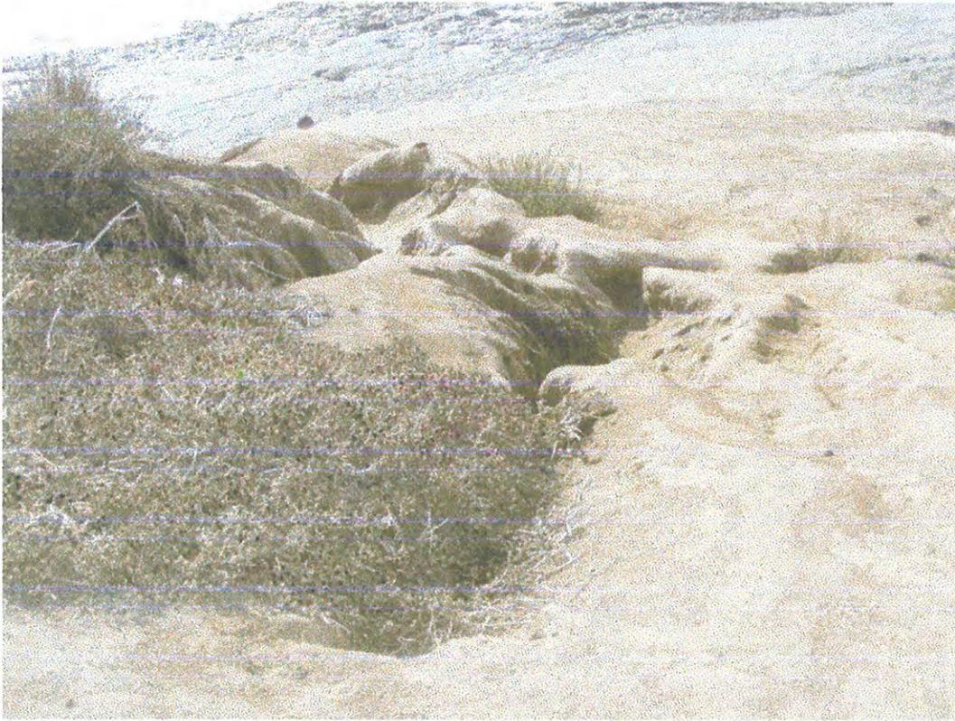
**Recommendation:** Install curbs around the parking lot to insure that all water from it drains towards Sunset Cliffs Boulevard. Scarify the soil and plant native vegetation on it to increase it's permeability and minimize seaward runoff.
