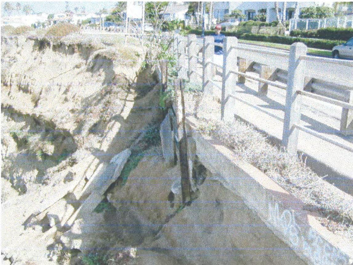
**Recommendation:** Continued monitoring of this area shown should be maintained to make sure that runoff doesn't run over the cliffs and further undercut the shoulder of the road and cause further cliff erosion. The erosion problems several hundred yards to the north needs to be investigated and action taken to prevent further cliff erosion.
