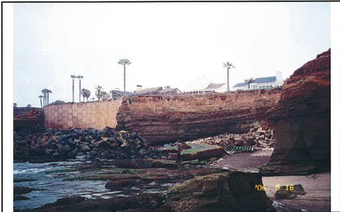
Figure 4B: MSE wall for bluff stabilization along with rip-rap at base near Adair Street. Terrace deposits of Bay Point Formation seen overlying Point Loma Formation.
