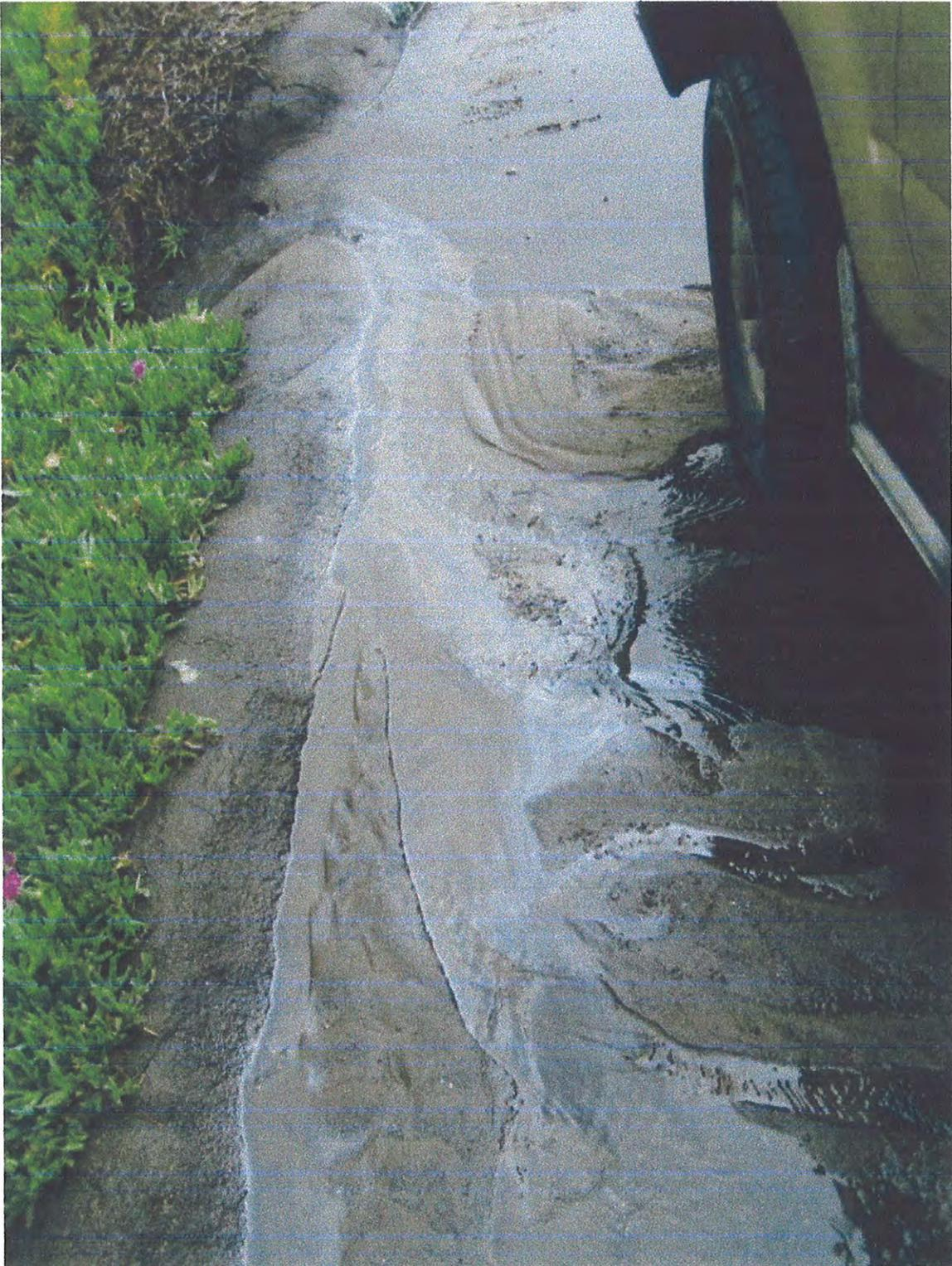
**Recommendation:** The runoff from the Upper Parking Lot should be captured by a surge dam or tank where it leaves the parking lot spillway, treated to remove contaminants, and
