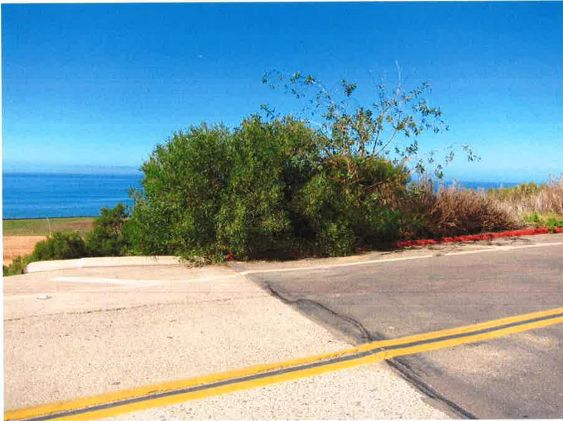
**Figure 24.** Due to low curb height at the northern edge of the Loop Road Arizona Crossing, runoff during moderate to high flow periods tends to flow around the northern edge of the Arizona Crossing apron and undermine it. The black Acacia branches cover the point where the runoff goes off the road.
