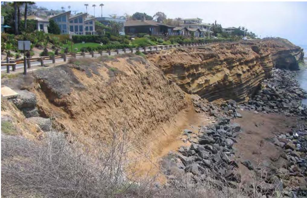
PH35: South of Monaco: No stratification along cliff face; The road was built on cove and filled it with rock and fill. The gabions need to go before they break and spill small rock all over the beach.
