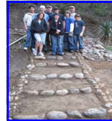
A Recent Eagle Scout Project. Because of a little ingenuity and a lot of sweat, this staircase may last forever.
