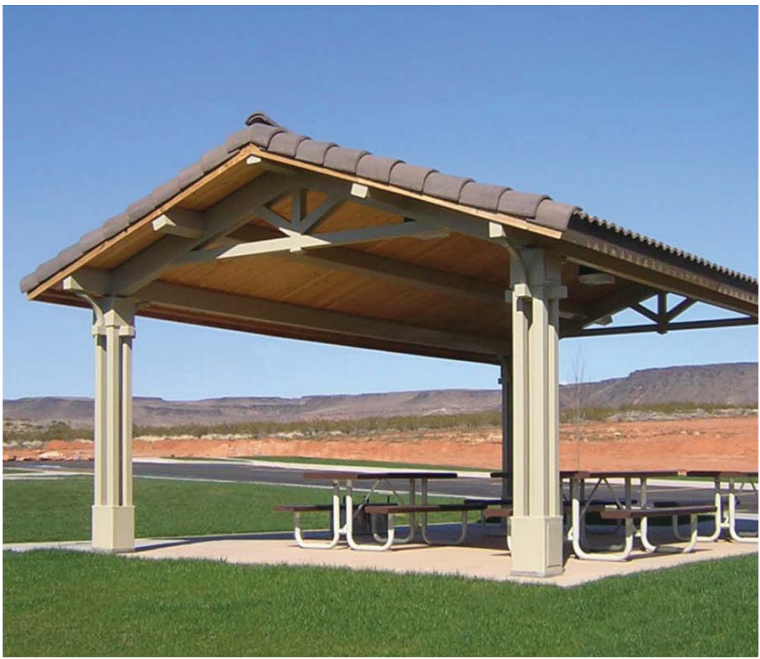
Prefabricated 16' x 36' steel structure with concrete tile roof to match restroom
