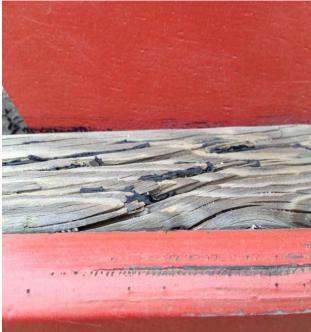
We observed a piece of wooden playground equipment, which, according to the PRD's Consultant Guide is prohibited. We rated the equipment as poor because of the raised wooden edges that could cause cuts, scrapes, and splinters.
