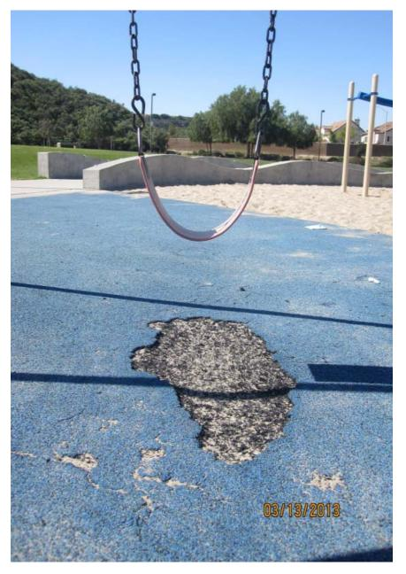
We rated this surface as poor because extreme cracking, ripping, or tearing was evident and the subsurface was exposed and trenched.
