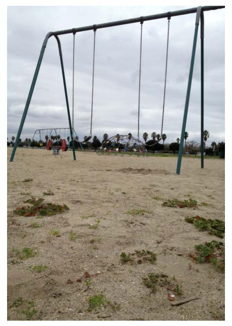
We rated the sand as poor because compaction and weeds were present.
