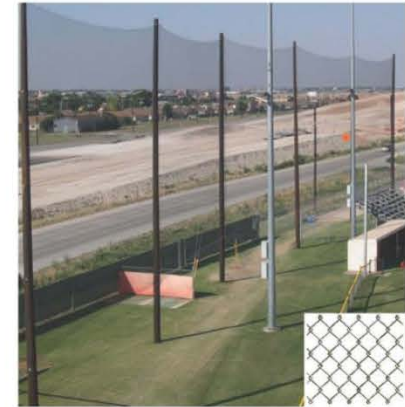
Barrier Fencing w/ Chainlink
