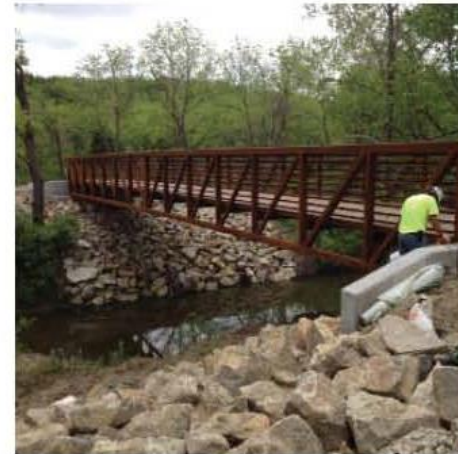
Weathered Steel Bridge
