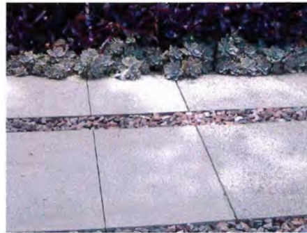
Concrete banding with decorative scoring pattern
