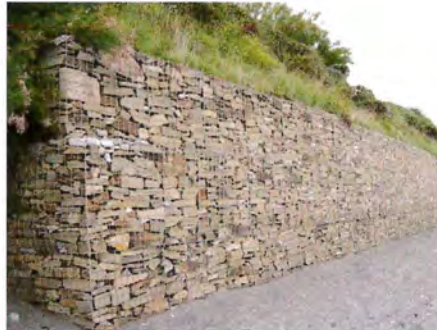
Gabbion wall (Type C)
