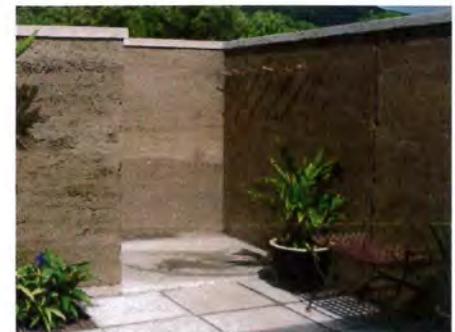
Rammed Earth (Type C)
