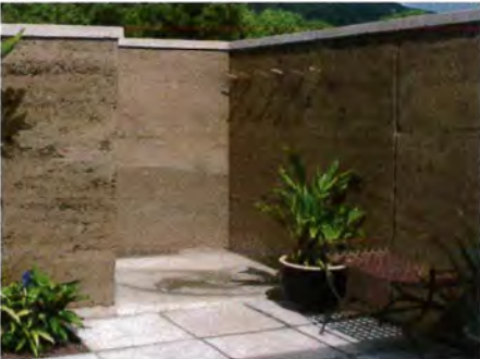
Rammed Earth (Type C)
