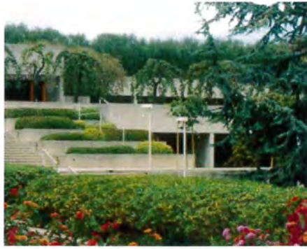
Use of retaining walls to create terraced landscape areas
