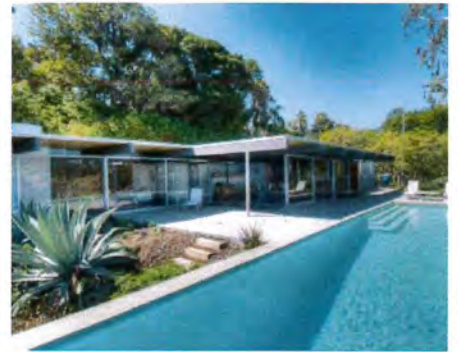
Project roof overhangs for shading
