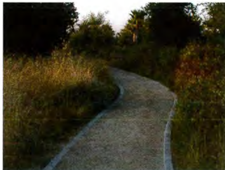
Stabilized decomposed granite
