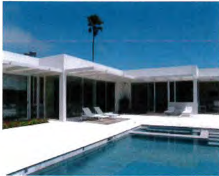
Project roof overhangs for shading
