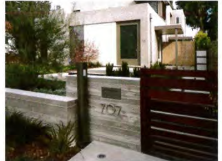
Board form concrete (Type B or C)
