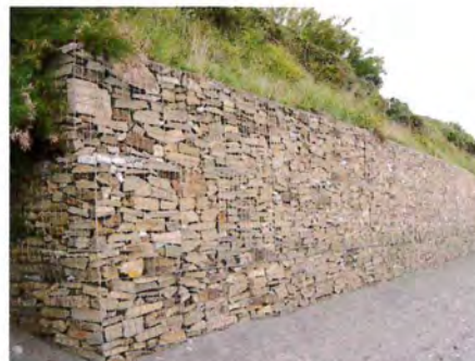
Gabbion wall (Type C)
