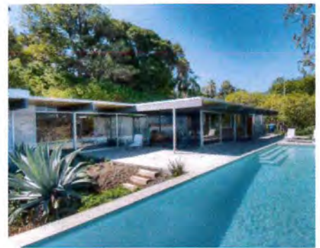
Project roof overhangs for shading
