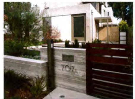
Board form concrete (Type B or C)
