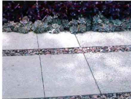
Concrete banding with decorative scoring pattern
