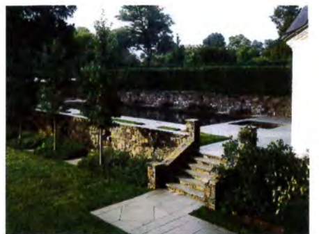
Use of retaining walls to create terraced landscape areas
