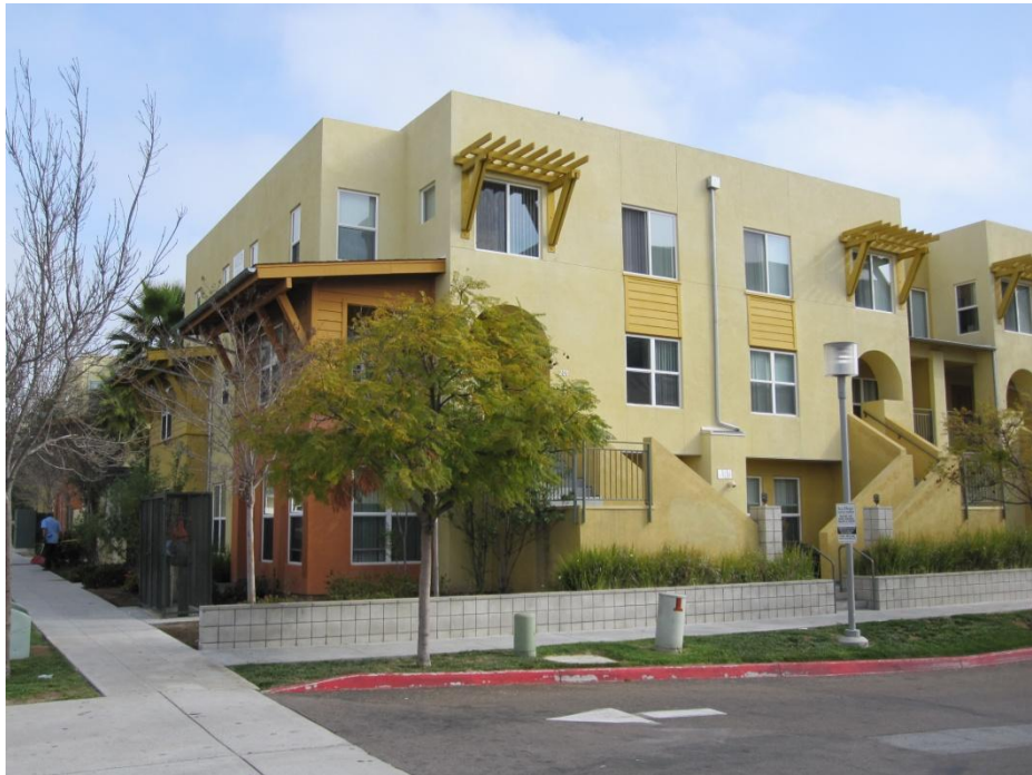
Affordable housing development north of University Avenue near Teralta Park. This photo illustrates the type of multi-family development that the City seeks to encourage within the study area and the surrounding Mid-City communities.
