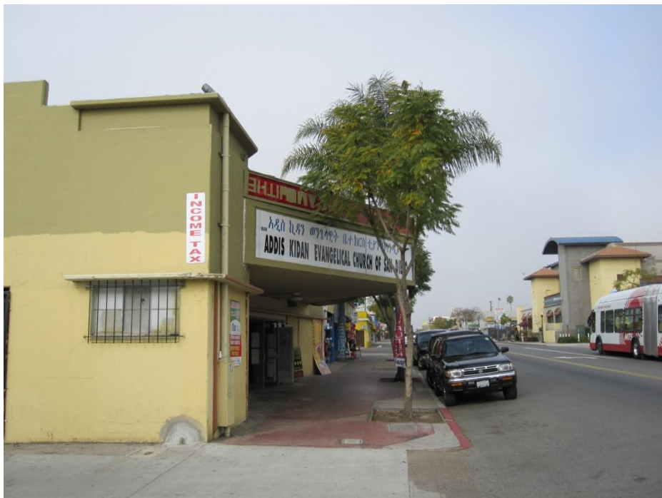
Commercial development in a converted movie theater along University Avenue. This photograph illustrates the type of older commercial development that characterizes parts of University Avenue and El Cajon Boulevard within the study area.
