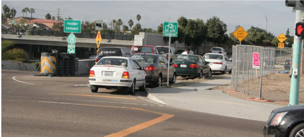
Image 7: Central Avenue becomes Terrace Drive. According to a plan for the SR-15 Bike Path forwarded to Randy Van Vleck by Caltrans Bike/Ped Coordinator Seth Cutter, Caltrans and the City intends are working to build a Bike Path from the Terrace Drive cul-de-sac to the south side of Adams Avenue and then from the north side of Adams Avenue to Mission Valley, as depicted in Images 7 and 8.
