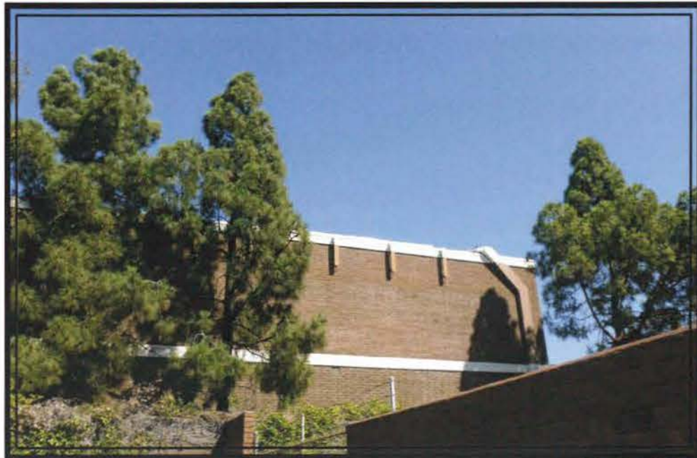
SITE PRIOR TO INSTALLATION
