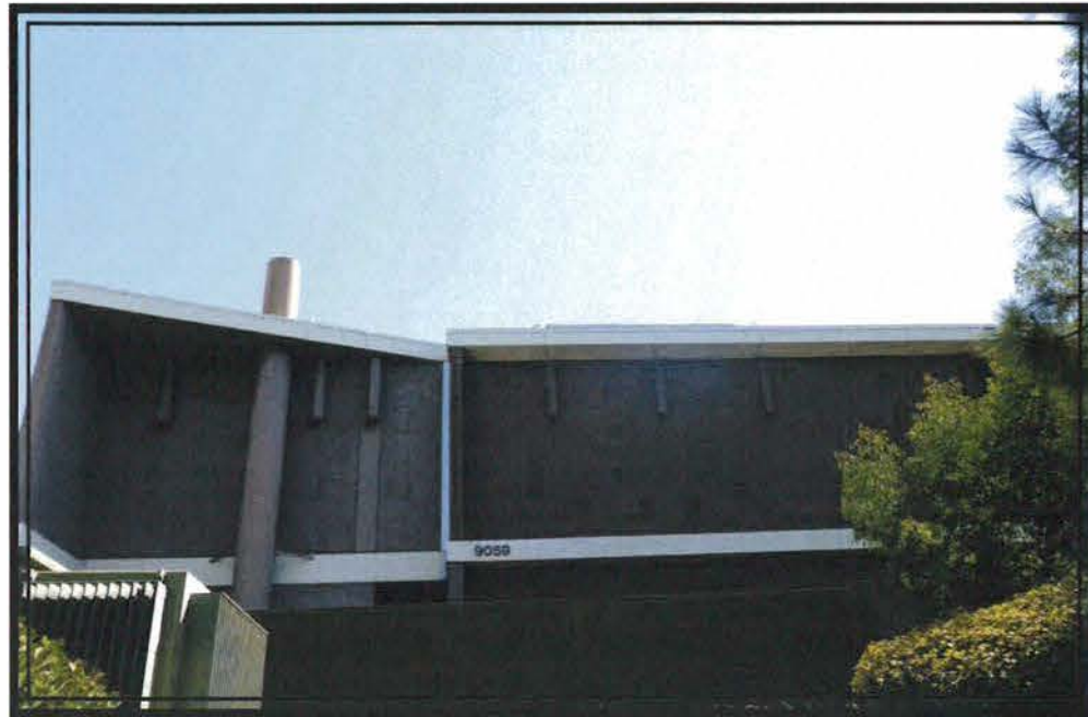
SITE PRIOR TO INSTALLATION
